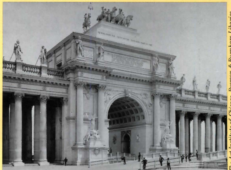
The Arch of Peristyle.
