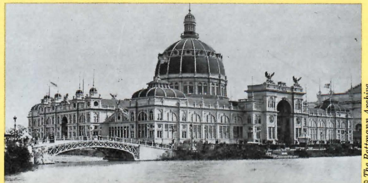
The U. S. Government Building, which Schuyler criticized in an "Architectural Aberrations" article.
