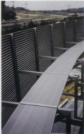
Screens made of metal strips block direct sunlight, but are low enough to maintain views.
