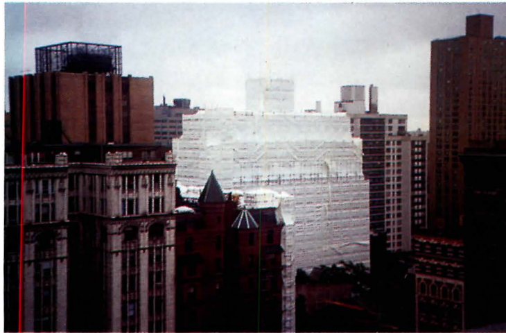
A steampipe explosion in New York City covered an apartment building with asbestos-contaminated mud.
