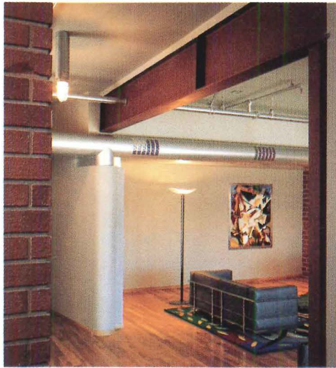
Hodgetts and Fung bridged time and space by revealing the old structure and inserting new elements in overlapping patterns. Plywood panels mimic original wood flooring (below), and Hodgetts and Fung's aluminum ducts weave through existing raw steel beams (above).
