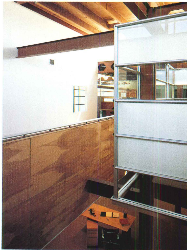
Hodgetts and Fung bridged time and space by revealing the old structure and inserting new elements in overlapping patterns. Plywood panels mimic original wood flooring (below), and Hodgetts and Fung's aluminum ducts weave through existing raw steel beams (above).
