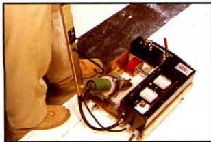
Self-propelled, hot-air welding machine fuses HyChoice seam.
