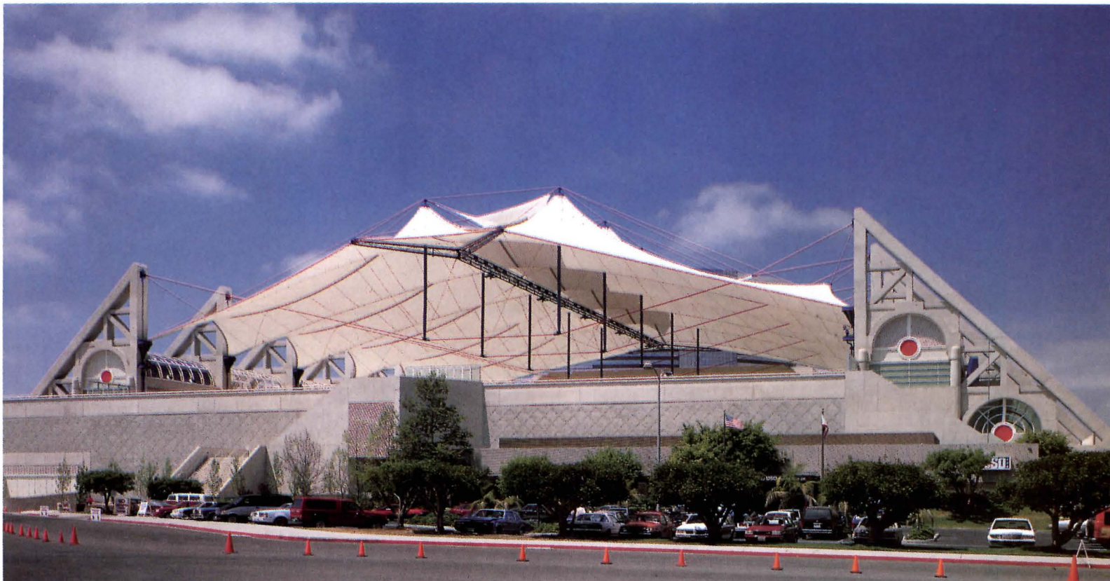
Above: the center meets Harbor Drive like an airline terminal. Below: tensile fabric roof covers an open-air exhibit deck.
