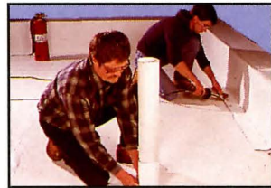
Roofing technician installing perimeter flashing and field-fabricated pipe-seals.
