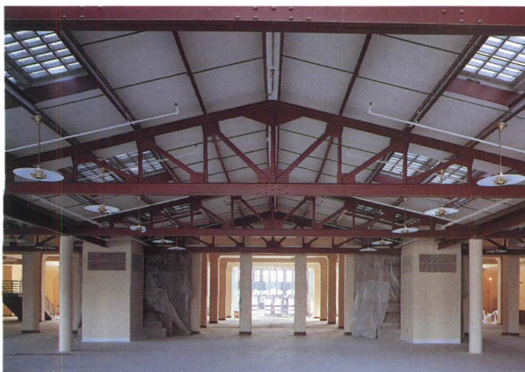
Roof of the Railroad Ticket Office has been rebuilt.
