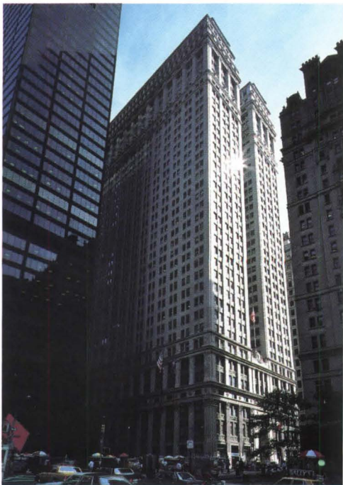
Drawings (right) were prepared from field surveys for remedial GFRP work at 120 Broadway (above).
