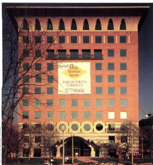
One Bowdoin Square's top-floor "cornice" is 39 panels of GFRC.
