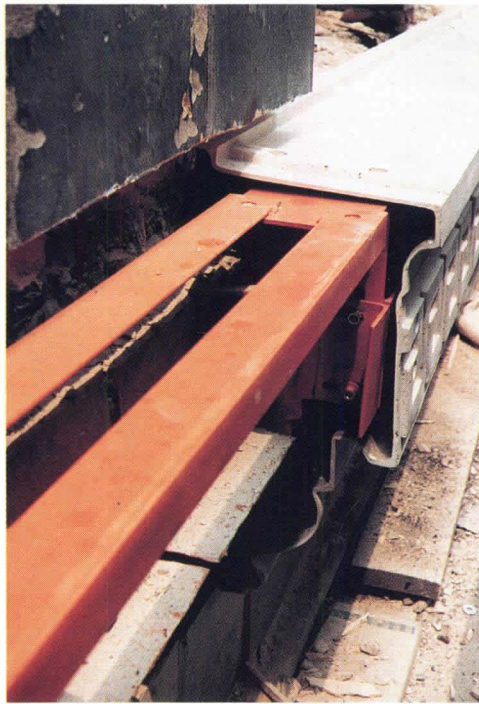
Steel brackets reinforce the GFRP and attach it to the structure.
