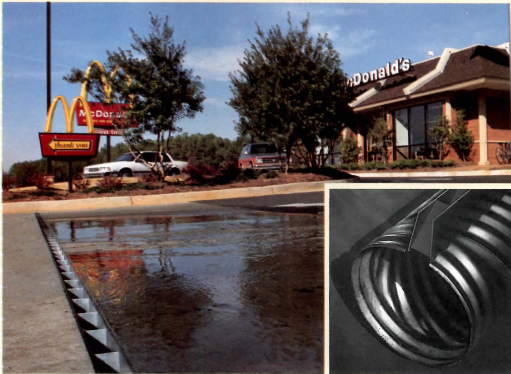
Contech Slotted Drain intercepts water from the parking lot before it can enter the street.
