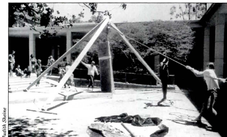
UCLA students reconstructed a section of the King's Road House using Schindler's innovative lift-slab technique (bottom photo). Schindler and his partner are shown building the original (top).
