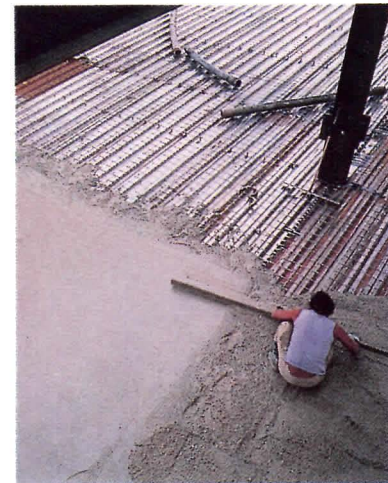
Composite deck simplifies construction
