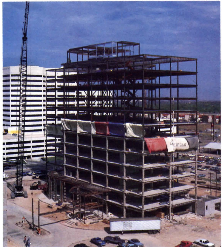
Vulcraft deliveries eliminated "lay down space" worries
