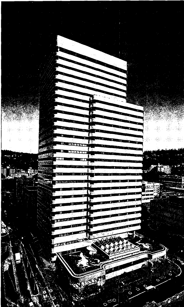
1. Pacwest Center, Portland, Oregon; The Stubbins Associates, Architects. A 735,000-square-foot mixed-use development in downtown Portland comprises a 30-story office tower, two floors of shops and restaurants along a through-block lobby arcade, and three levels of below-grade parking. Clad in alternating bands of anodized aluminum and silver reflective glass, the tower consists of two interlocking rectangles stepped back to permit a roof garden on the 25th floor. At ground level widened sidewalks, covered pedestrian walkways, brick paving, granite curbs, and a variety of street furnishings reinforce the character of Portland's existing transit mall.
