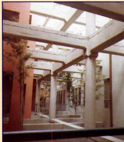
Atriums were created to achieve open air areas as well as apartment access. Note the size of the 1906 concrete beams.
