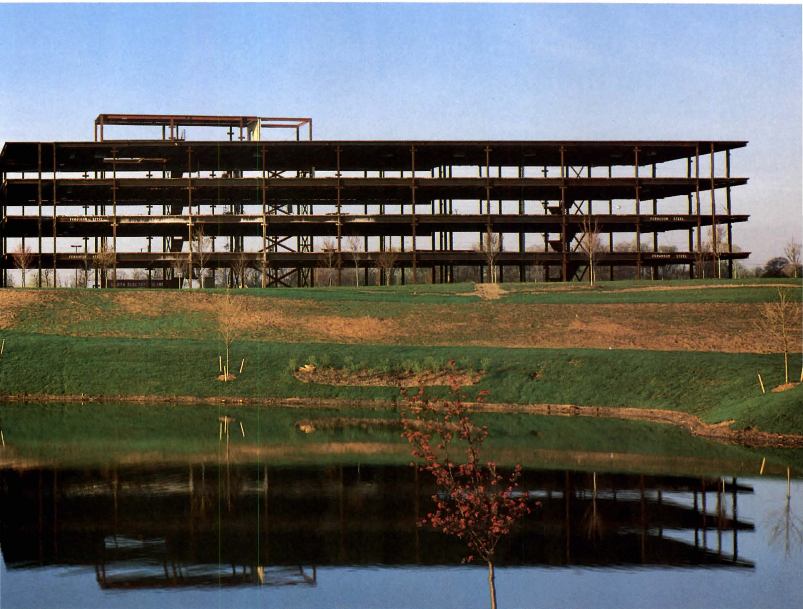
The Woodfield at The Crossing office complex in Indianapolis used 216 tons of Vulcraft joists and 169,000 sq. ft. of Vulcraft steel deck.
