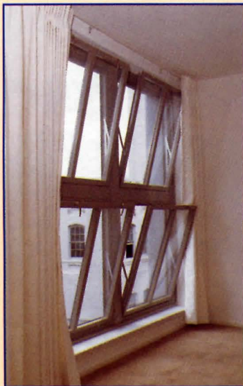
Exterior windows tilt in for easy cleaning. Heavy duty architectural windows with insulating glass preserve the historical feeling of this building.
