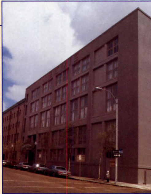
Bemis Bag Warehouse, built in 1906, is the first poured concrete building in Louisiana. Today it is Julia Place, 110 apartments located in downtown New Orleans. It's another historical building preserved by Alenco.
