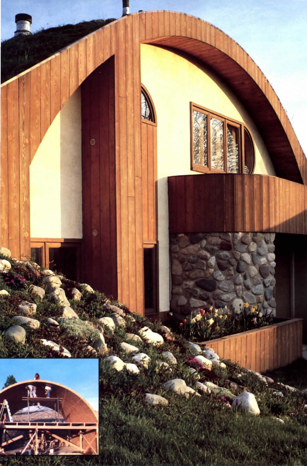
This earth covered arch home was designed by John Loveless and Jeremy Berg, IBS, Grand Haven, Michigan. The 38-foot span of arch is self-supporting and constructed of foam core panels made with Weyerhaeuser Structurwood skins.
