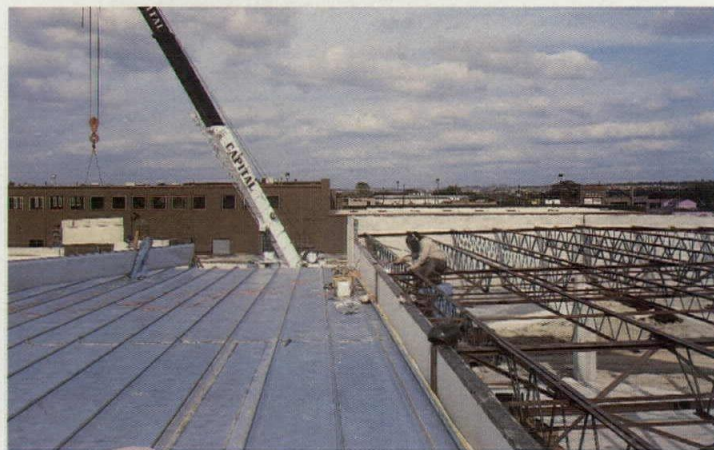
Vulcraft standing seam roof with joists and joist girders.
