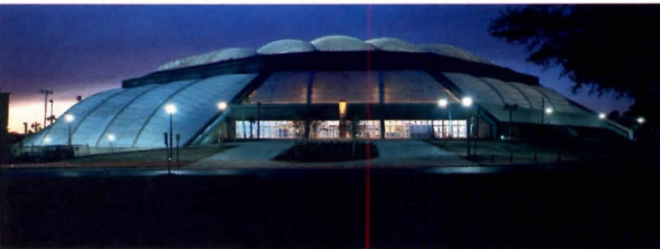
1. AN/6B Radome, United States Air Force, Cornell Aeronautical Laboratory; engineer: Walter W. Bird. 2.,3. Stephen C. O'Connell Center for Student Activities, University of Florida, Gainesville; CRS Serrine Architecture—Paul Kennon, design principal; structural engineer: Geiger Berger.
