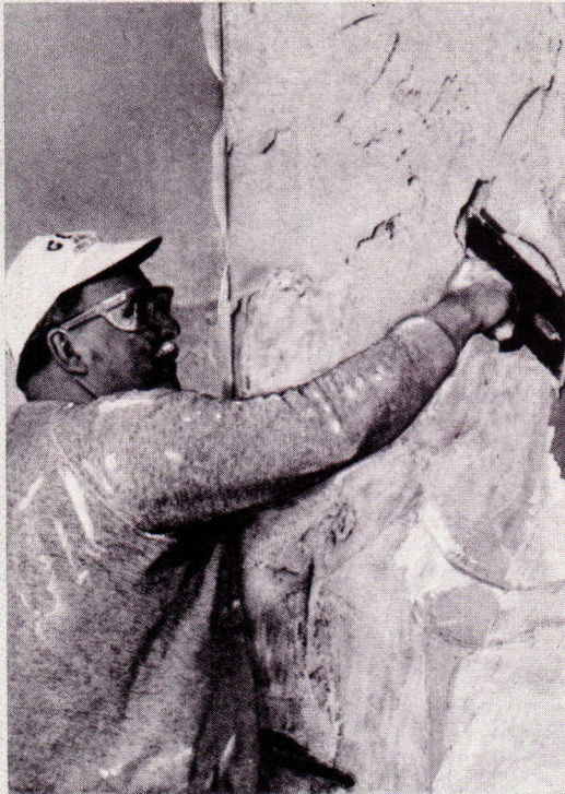
BEST WAY. Portland cement mortar over lath was great when labor costs and time delays were acceptable.
