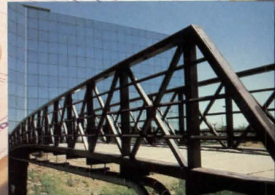
Denver, CO - Tamarack Square
