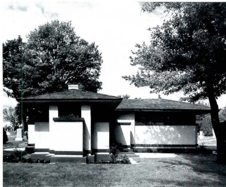
This small 1905 funeral chapel, Frank Lloyd Wright's only venture in the genre, recovered from the bedraggled state seen at right. Repair of the original pale green stucco called for filling in windows at ground level that lighted a basement excavated after construction. Solid doors on each side of the front steps were glazed (top) per the original design.
