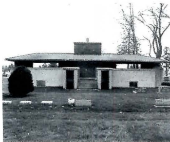
This small 1905 funeral chapel, Frank Lloyd Wright's only venture in the genre, recovered from the bedraggled state seen at right. Repair of the original pale green stucco called for filling in windows at ground level that lighted a basement excavated after construction. Solid doors on each side of the front steps were glazed (top) per the original design.
