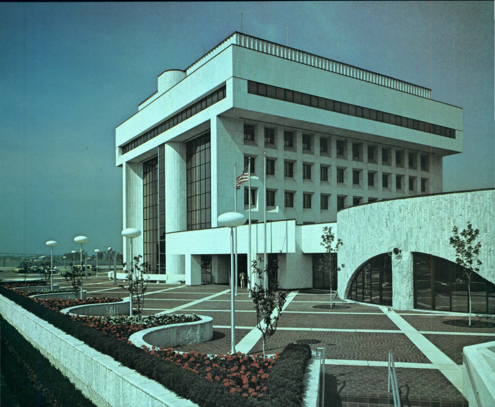
Port Huron Municipal Office Center Building, Port Huron, Michigan | Arch: Richard C. Cogley | All white material in photo is Cherokee marble, supplied by Genesee Cut Stone & Marble Co., Flint, Michigan
