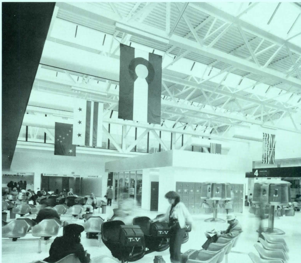
Spanning the terminal concourse of Buffalo's Metropolitan Transportation Center is a series of exposed steel trusses, 140 feet long, and these are cantilevered outside for covered access to the buses. A series of skylights, running above the trusses, admit lots of natural light, dappling the interior with plentiful, changing moods. A roof garden, on the second level, overlooks this busy room, creating a spatial hinge between the horizontal element of the concourse and the vertical element of the adjacent office building. Views south take in the city's rich architectural heritage.
