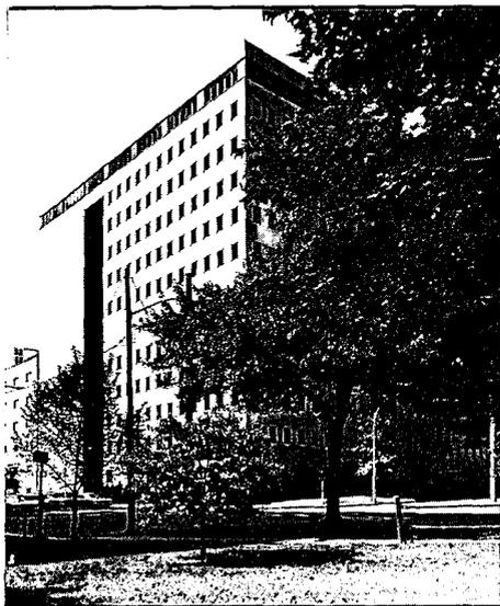
Almost 1,000 Aztec low temperature electric radiant ceiling panels were specified to provide perimeter heat along cold walls to supplement the heat generated by equipment, lights and people in an energy saving system especially designed for the AT&T Long Lines building at White Plains, N.Y.
