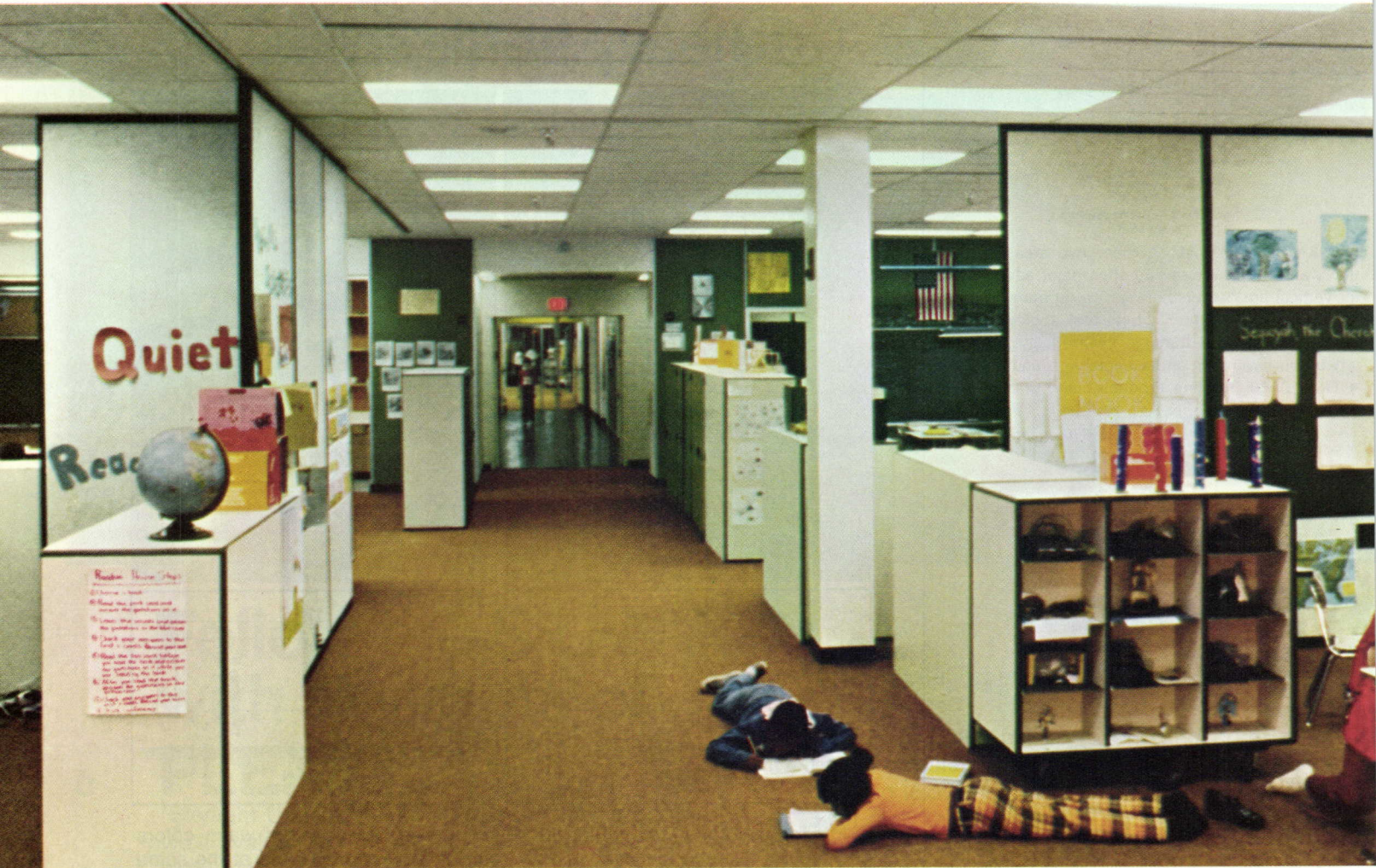
Same corridor after permanent, non-load bearing walls were removed. Placement of panels creates teaching clusters; tackable surfaces serve as teaching tools. Fletcher-Thompson Inc.—Bridgeport, Ct., architects/engineers.
