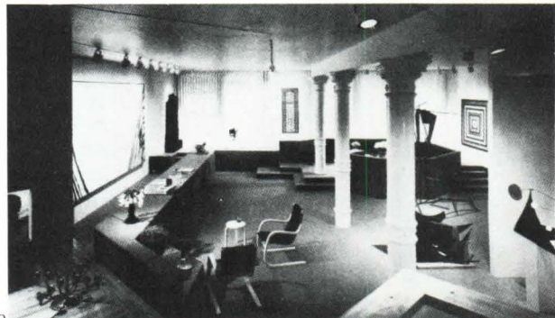
60 Loft restoration, Soho, New York City; Hanford Yang, architect; August 1975.
