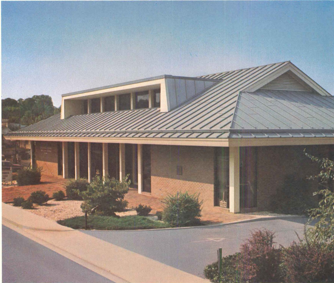
Greenville Federal Savings and Loan, Greenville, Tenn., Architect: Boyd & Arthur
