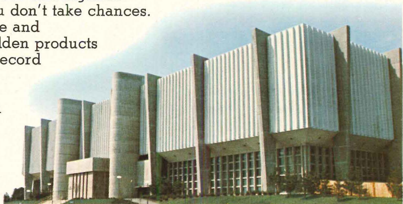
The Coliseum, 2923 Streetsboro Road, Richfield, Ohio
