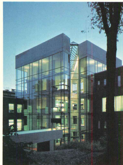
At the point at which the chemistry building and the physics building are linked by the tower, a broad entrance staircase has been created. The interconnecting floors can be seen through the glass facade. At night (below) the lighted tower becomes a landmark.
