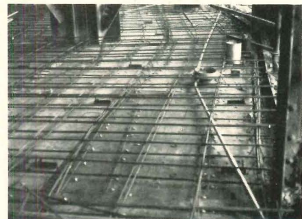
Galvanized rebars under surface of decking.
