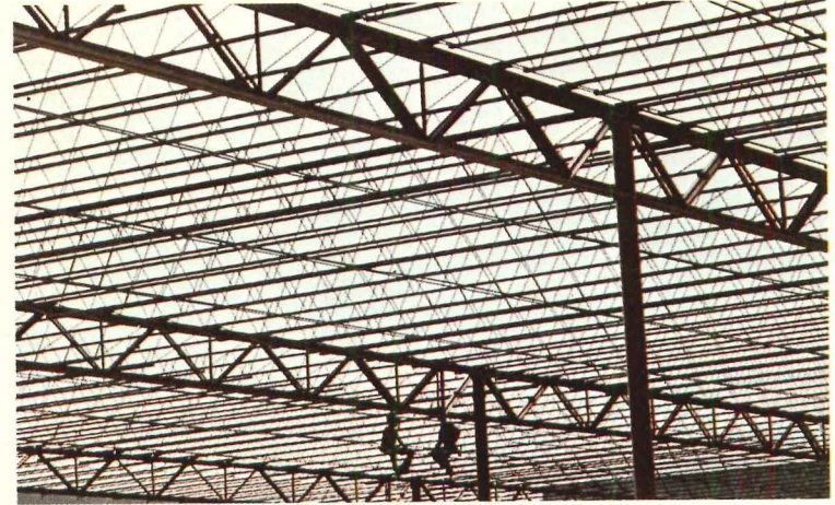
717 tons of joists and 433 tons of joist girders were used in this 746,852 square foot job.
