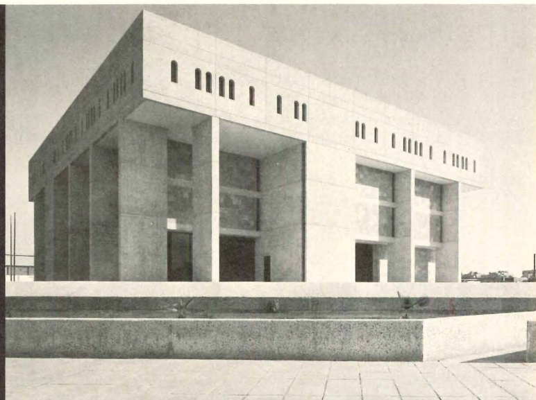
Emphasizing the necessity for on-site control of construction, the architects TAC for the Kuwait Fund Building (above) and Rader Mileto for the Horsemanship Club in Riyadh (below) are producing successful, finished products—despite construction limitations (see next page).
