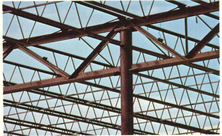
Lighter weight columns can oftentimes be used with joist girders. And that's a big advantage.
