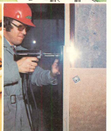
STRUCTO-GARD , protects columns from fire for one hour.
