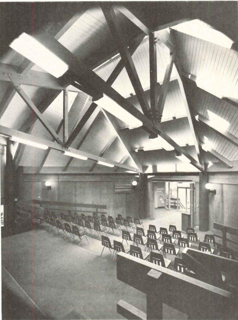
The dramatic roof of this auditorium covers the interstitial space which in other modules is a courtyard between classroom, lab or office facilities. The complexity of the roof structure offsets the simplicity of the other buildings, prefabricated entirely and erected on the site in a three-month period. The college will eventually serve 1000 students, three-fourths of whom are drawn from the Oakland area. Privately-built housing adjacent to the campus provides for out-of-area students. 1. Top of auditorium roof is visible from cluster of modules. 2, 3. Auditorium. 4. Corridor.
