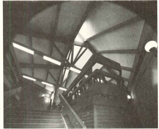
The dramatic roof of this auditorium covers the interstitial space which in other modules is a courtyard between classroom, lab or office facilities. The complexity of the roof structure offsets the simplicity of the other buildings, prefabricated entirely and erected on the site in a three-month period. The college will eventually serve 1000 students, three-fourths of whom are drawn from the Oakland area. Privately-built housing adjacent to the campus provides for out-of-area students. 1. Top of auditorium roof is visible from cluster of modules. 2, 3. Auditorium. 4. Corridor.
