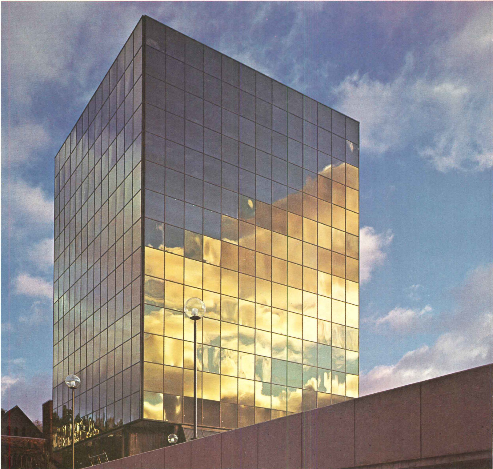
Owners: Detroit & Northern Savings & Loan Assoc.; Architect: Maurice B. Allen, Jr., A.I.A., Tarapata-MacMahon-Paulsen Corp., Bloomfield Hills, Michigan
