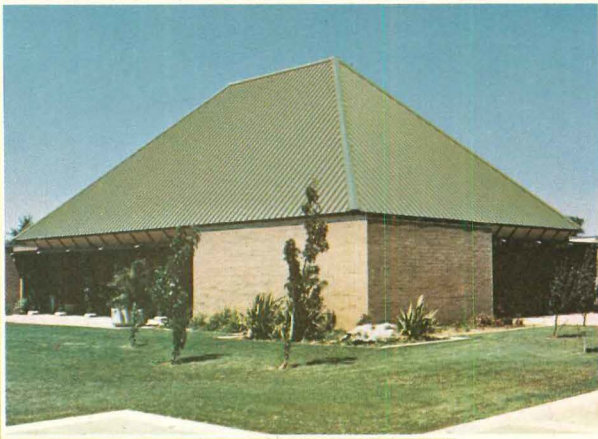
An attractive, tight hip roof.
