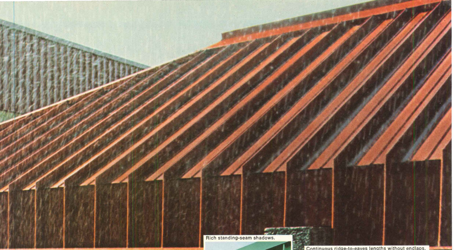
Continuous ridge-to-eaves lengths without endlaps.
