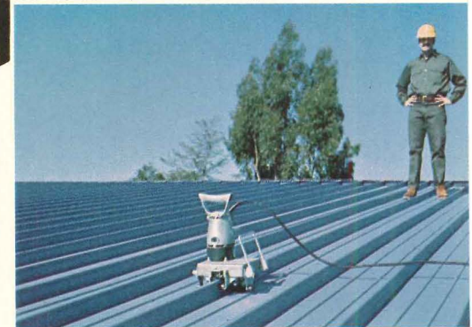
Closure tool "zips" the seams tight.
