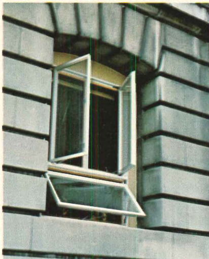
Renovations to Kenton, Ohio, Hardin County Courthouse for Hardin County Board of Commissioners.
