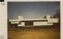
wide. Standard shell construction features an extruded aluminum or steel frame. Standard 1/4-in. glass is used. The roof is equipped with a water control system. / Ventaire Corp. A,I\*
