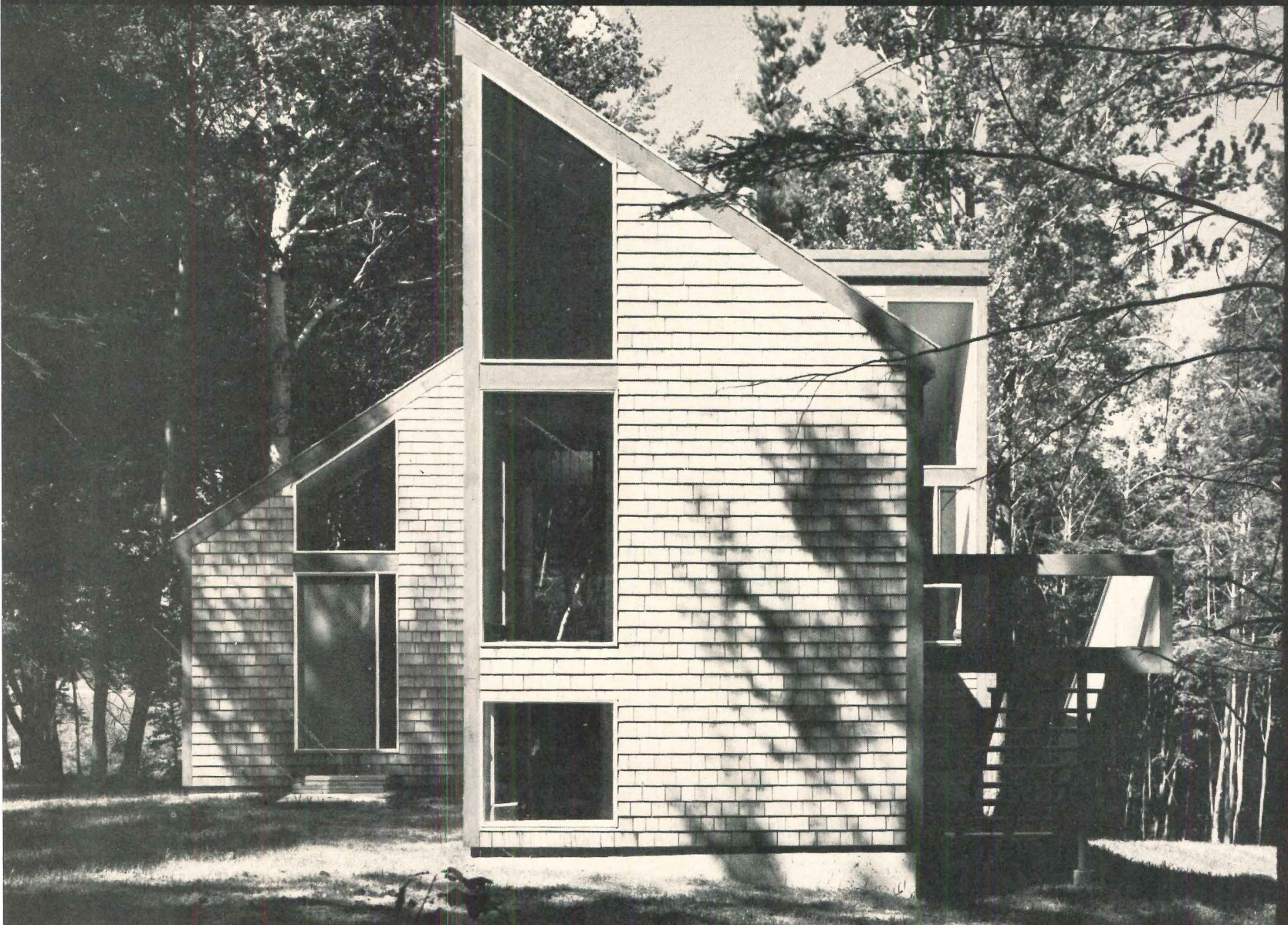
Vacation home at Francestown, New Hampshire. Certigrade Shingles No. 1 Grade 16" Fivex. Architect: Brett Donham.
