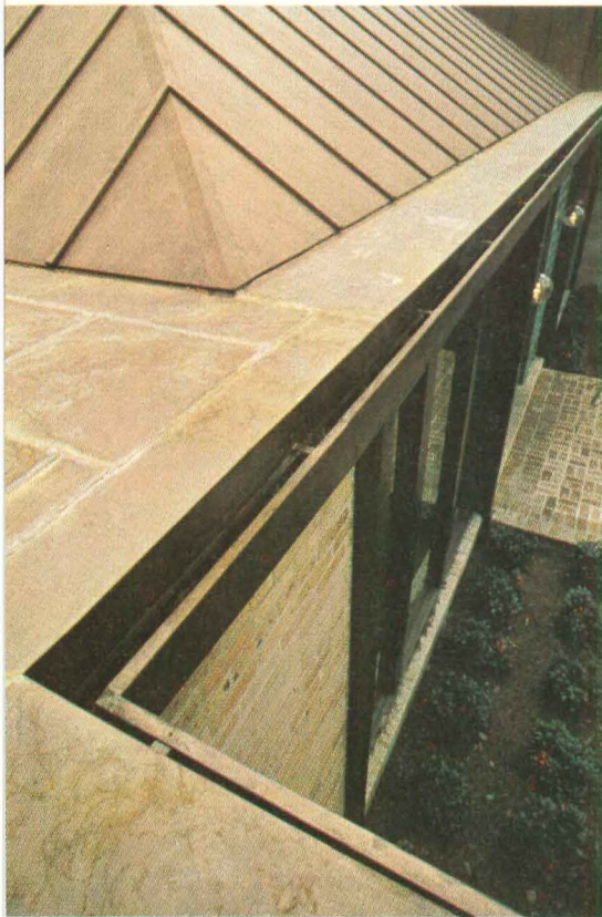
Copper gutters and flat roofing (above). Corrosion-resistant copper is as functional as it is beautiful. Highlights quality.
