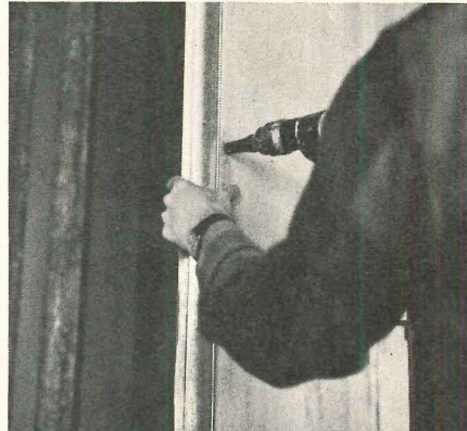
3. Attaching core to T-spline.
