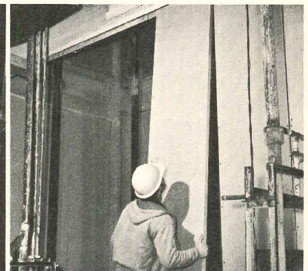
2. Installing core panel.
