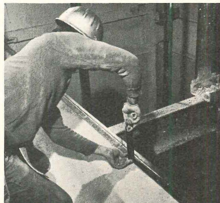
1. Installing floor track.
