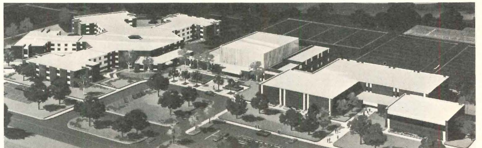
Architect: Owen F. Hackett, Jr. & Associates, New Bedford, Mass. Structural Engineer: MacLellan, Dormer, Mulcahy, Inc., Providence, R.I. General Contractor: Perini Corp., Framingham, Mass.
