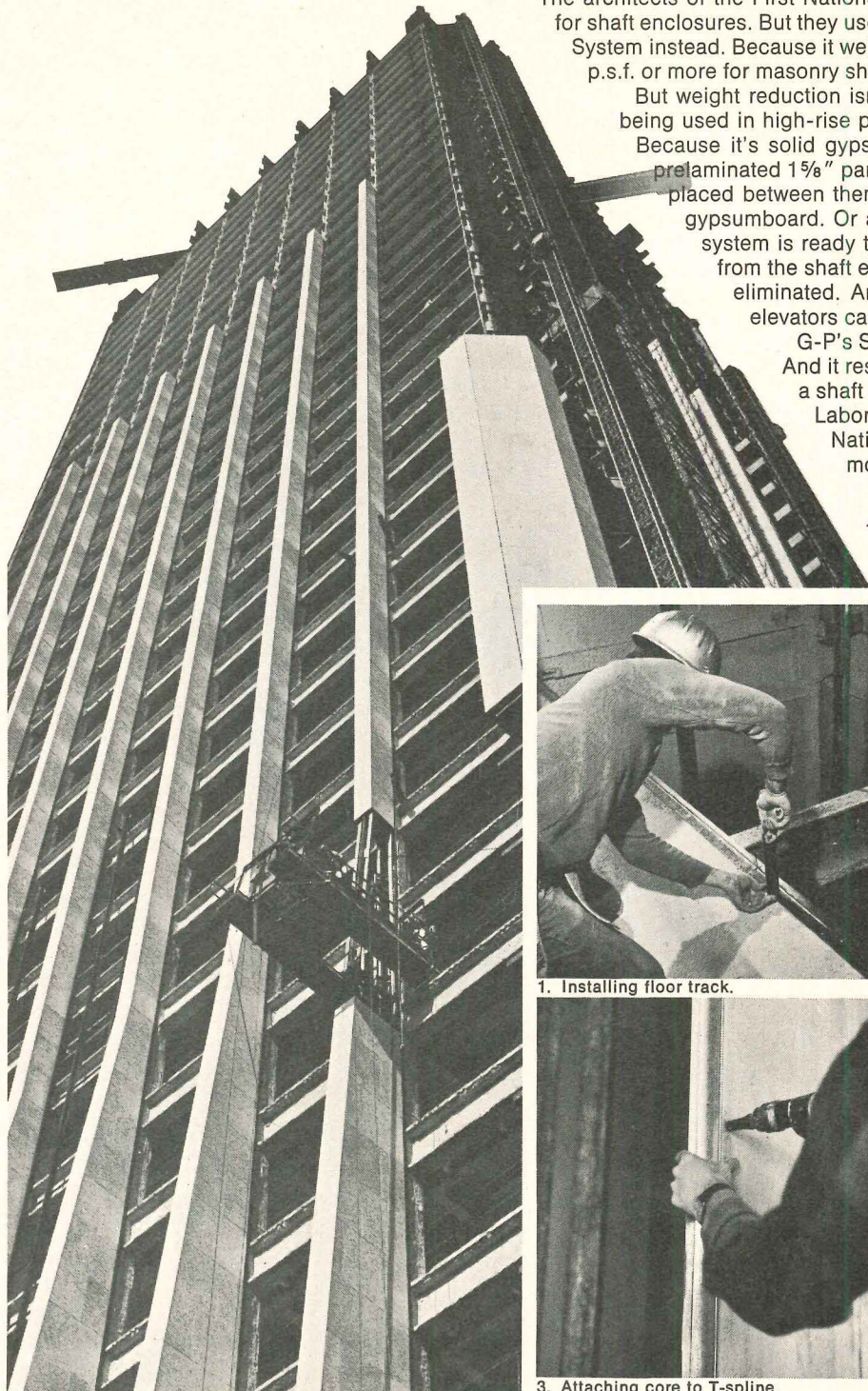
3. Attaching core to T-spline.
