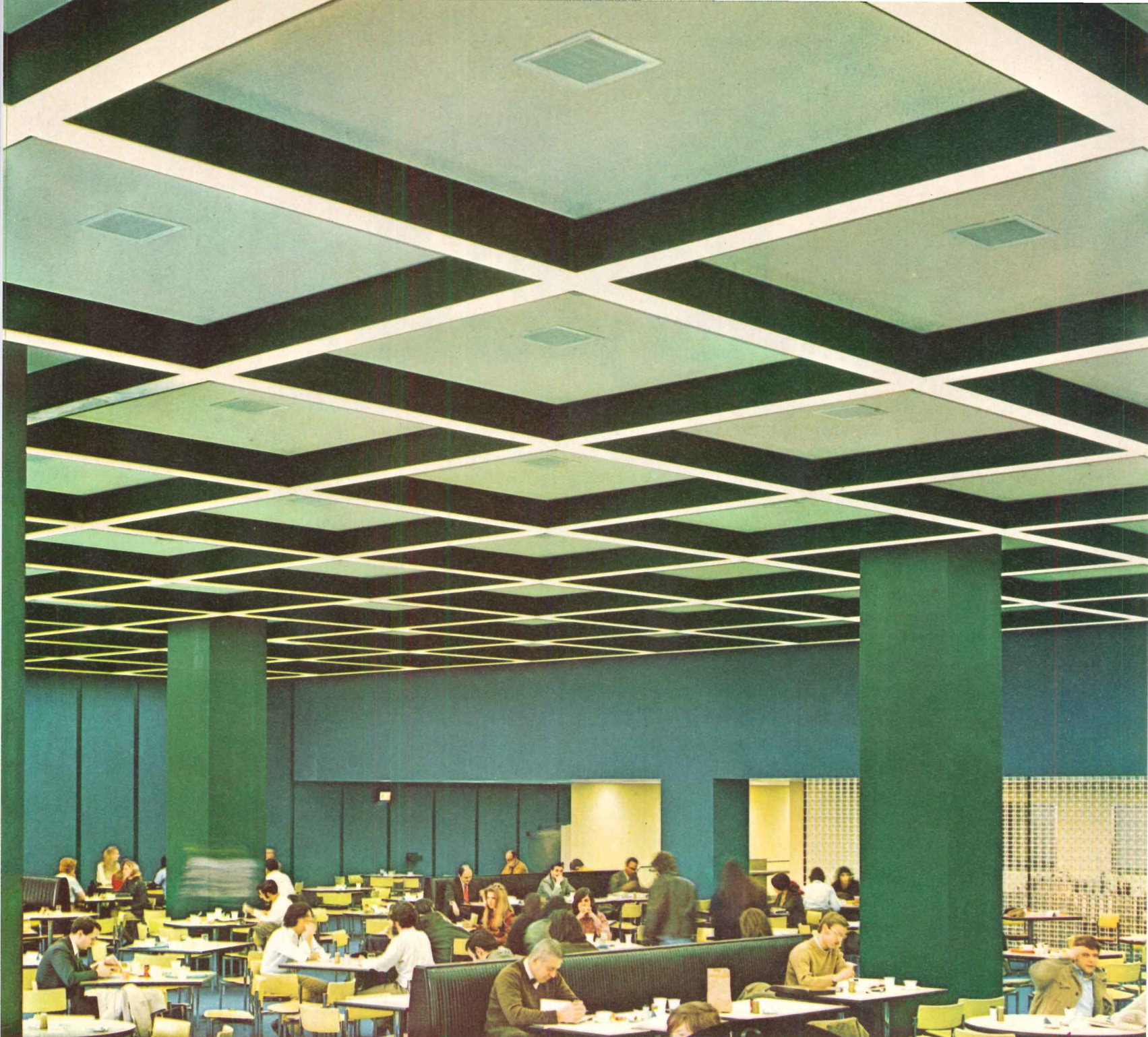
University Center of George Washington University. Unusual ceiling beam lighting fixtures custom-engineered by Keene Sechrist Lighting, working closely with Syska & Hennessy, Inc., the project engineering firm. Architect: Mills, Petticord & Mills.
