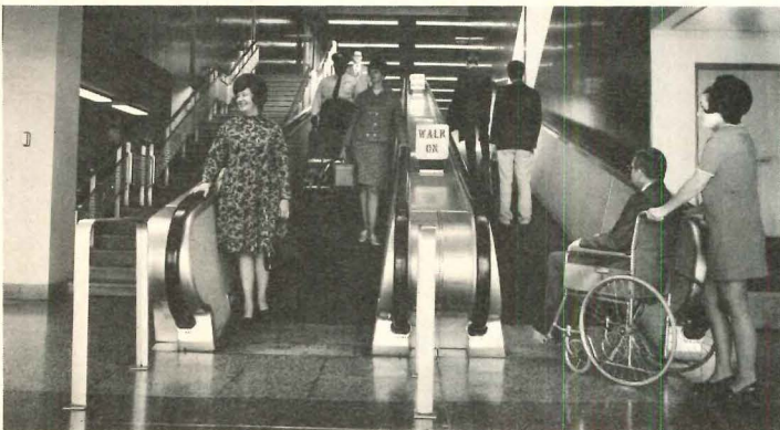
SPEEDRAMP incline belt passenger conveyor
