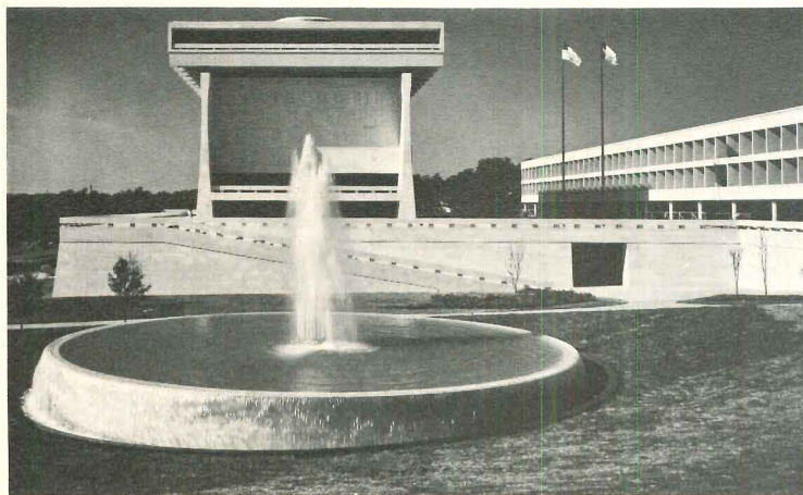
The Lyndon Baines Johnson Library , University of Texas, Austin, Skidmore, Owings & Merrill, Brooks, Barr, Graeber & White, architects, is becoming known as Lyndon's Pyramid. The combined museum and library is an eight-story monolithic structure with an 85 ft square and 55 ft high Great Hall with one glass wall exposing five levels of archives.
