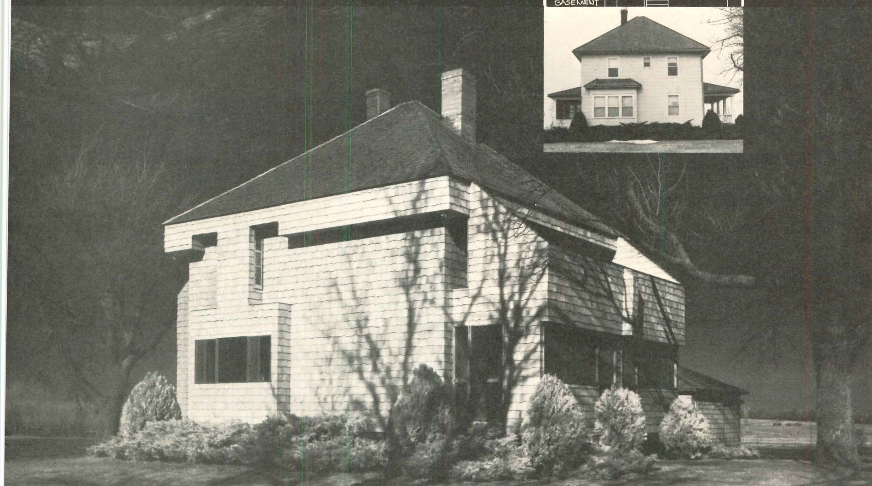
Residence at Gardner, Kansas. Certigrade Shingles No. 1 Grade: roof, 24" Royals; walls, 16" Fivex. Architects: Seligson/Egger. Owner-contractor: Henry McGrew.
