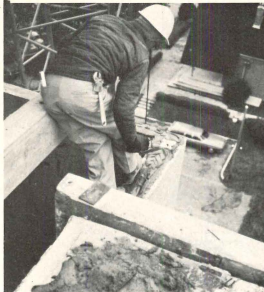
8. Troweling grout prior to setting next core unit
