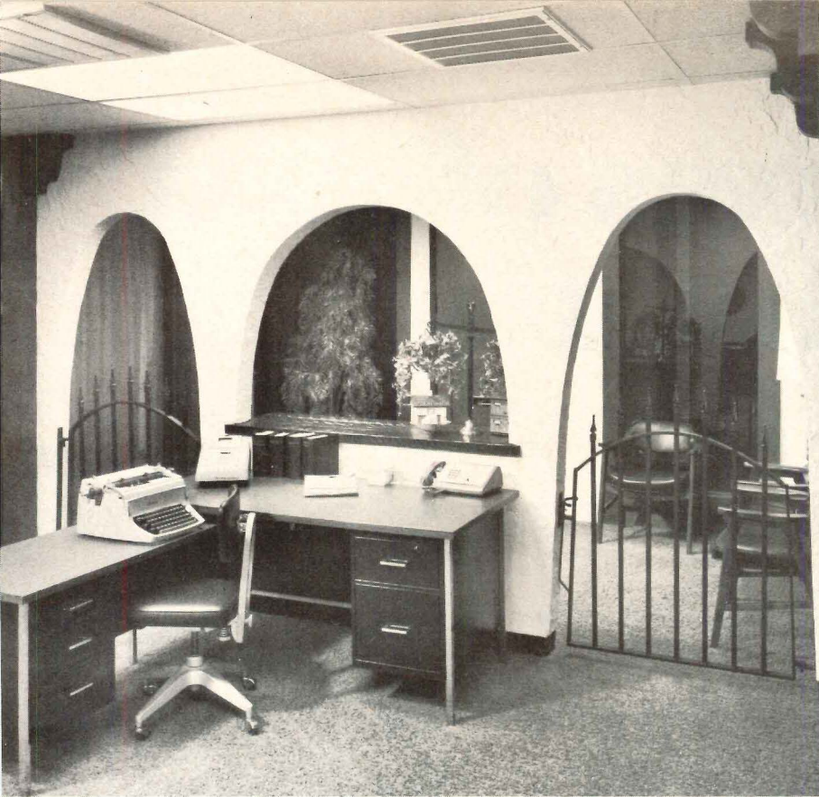
Tulsa's 2800 Center Building is heated and cooled by 50 Lennox blower-coil-filter units with resistance electric heating and . . .
