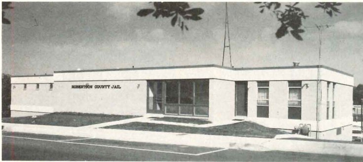
Diversity of building types and inter-state distribution of practice characterizes the Yearwood & Johnson pattern. In addition to the substantial backup of the education division in their schoolwork, the firm gives equal attention to such
