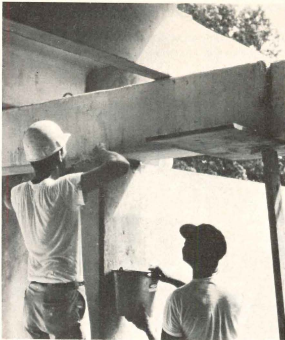
7. Placing epoxy grout between beam and core
