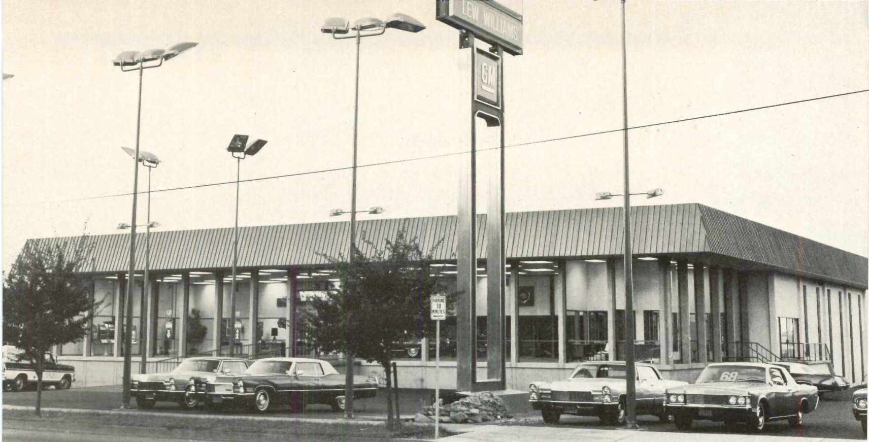
Lew Williams Cadillac, in Portland, Oregon, uses a Lennox roof mounted, gas-electric, single package air conditioner to heat and cool this showroom and office.
