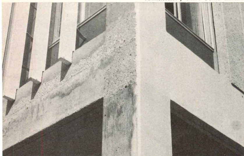
G. section of building—before and after
