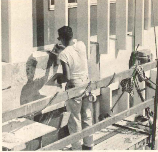
B. leveling the sills
