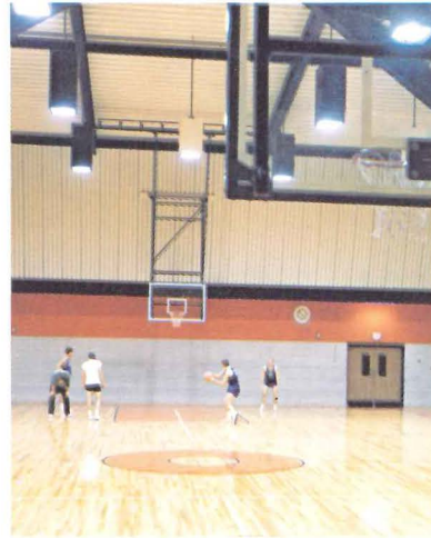
Twenty Spectra VI pendants provide an average 81 footcandles of uniform lighting in this gym. These rugged but handsome fixtures are available in 400 and 1000 watt models.
