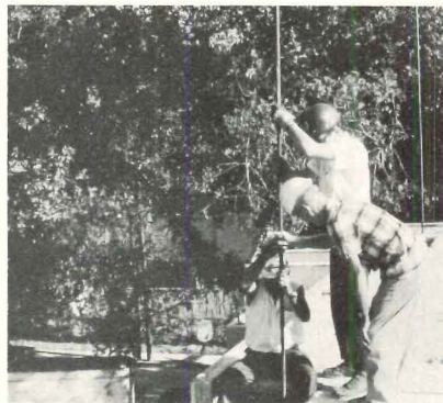
10, 11. Post-tensioning of core units
