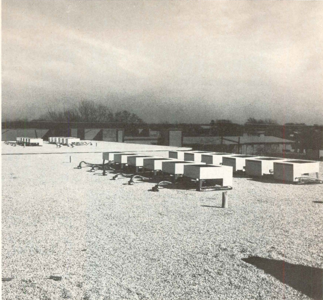
Mi Amigo Apartments, under construction in Dallas, is a complex of 149 apartments with individual ducted Lennox heating and air conditioning. New-design cooling units hide low on the rooftops. Architect: John Moss. Building Contractor: GTC Company. Heating/cooling contractor: Citywide Plumbing & Air Conditioning. Owners: George T. Connell and M. I. Harris, Jr.
