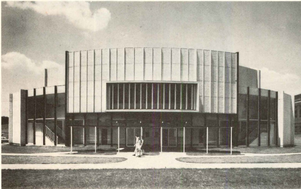
Theater and Classroom Building, Birmingham-Southern College, Birmingham, Ala. Architects: Warren, Knight & Davis. Theater Consultant: Dr. Arnold Powell. General Contractor: Brice Building Company, Inc. Dover Stage Lift installed by Dover Elevator Co., Atlanta.
