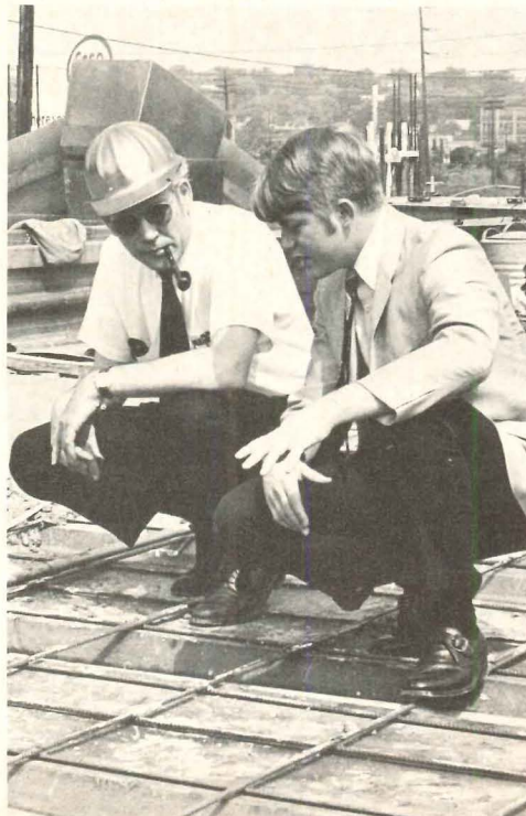
Student Vance W. Travis (below) looks over plans with Ken West, head of the construction department of Earl Swensson and Associates of Nashville, then (right) goes with Ken to check conditions at the site.
