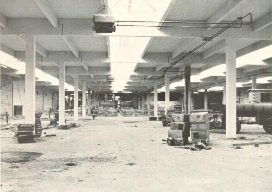
The one-story production layout plan of the factory was provided by Rosenthal. A complete precast structural system was devised which integrates the need for plan flexibility on a 30-foot bay. The system allows the building, including skylights and
