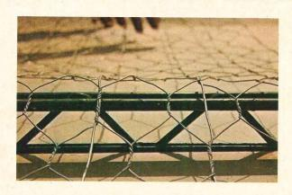
Open webs of Keydeck subpurlins permit the polyurethane foam to form a monolithic sheet. Keydeck reinforcement rolls out flat and easy.
