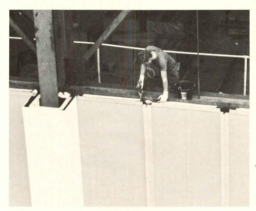
Mammoth-size high-voltage laboratory is sheathed in metal-faced sandwich panels having a 5-in. core of foamed polyurethane. Skins are separated by vinyl ties which also serve to join one panel to an adjacent one. Metal skins serve as an electronic shield. Joints between panels are foam-filled in the field.
