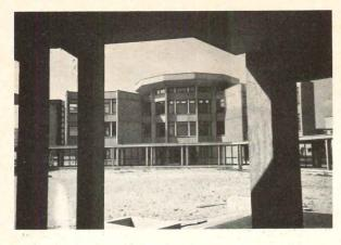
The eight individual buildings of the main school complex will be connected with glazed-in walkways which can be seen in the photo at left. All buildings are built in reinforced concrete poured in situ.
