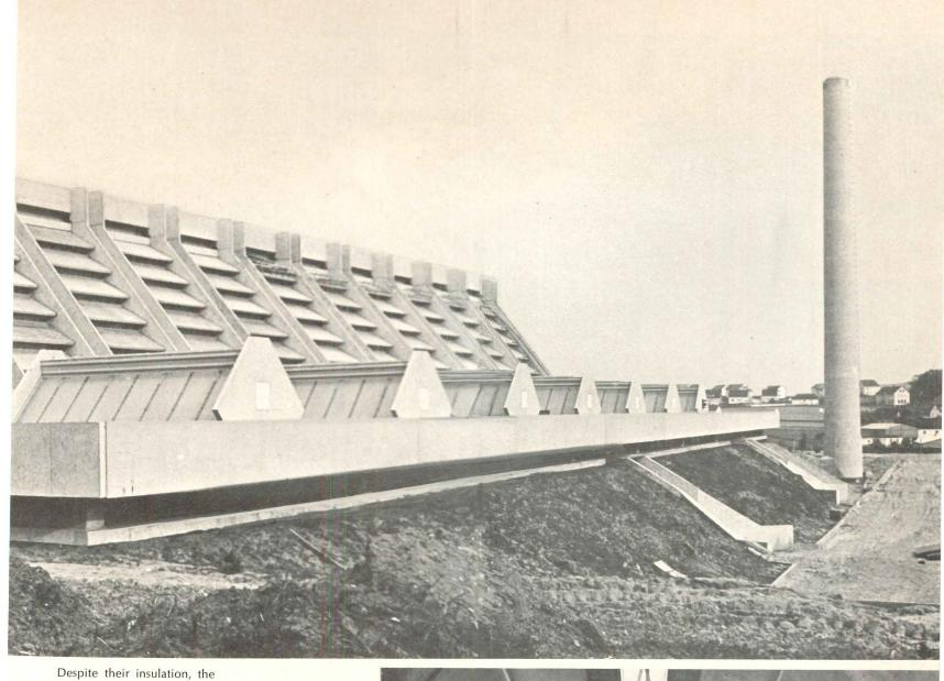
glass ovens give off great quantities of heat, and the glass is worked in the open at temperatures from 1292°-2372° Fahrenheit. Gropius and his TAC colleagues solved the problem of drawing off the excessive heat without the aid of special air conditioners. As the heat rises and exhausts between the louvers, cool air is drawn in through the inner courtyards shown in the plan and section (left). The interior photograph (right) was made before the glass ovens were installed.
