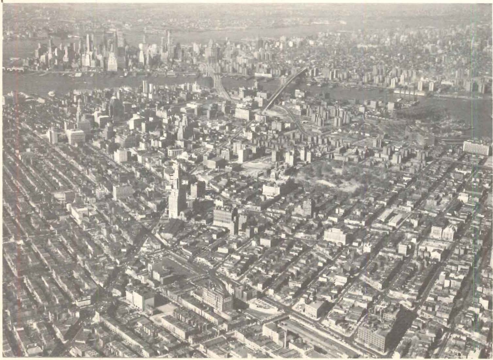
The area is on axis with the major bridges to Manhattan.
