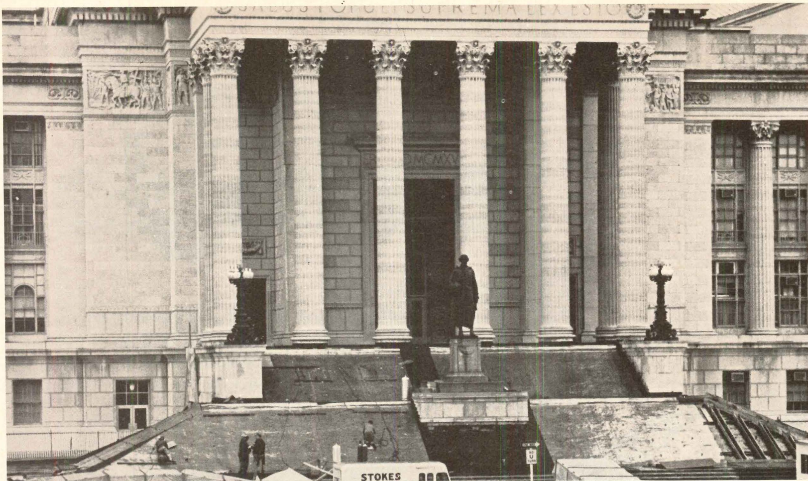
Architect: Bernard McMahon, Clayton, Mo. selected by the Missouri State Board of Public Buildings—Gov. Warren E. Hearnes, Chairman, Lt. Gov. Thomas F. Eagleton, Secty., Attny. Gen. Norman H. Anderson, Member, under direction of Div. of Planning and Construction, John D. Paulus, Jr., A.I.A., Director. General Contractor: E. G. Linhardt Constr. Co., Jefferson City, Mo. Lead Sub-Contractor: Larry Goad & Co., St. Louis.
