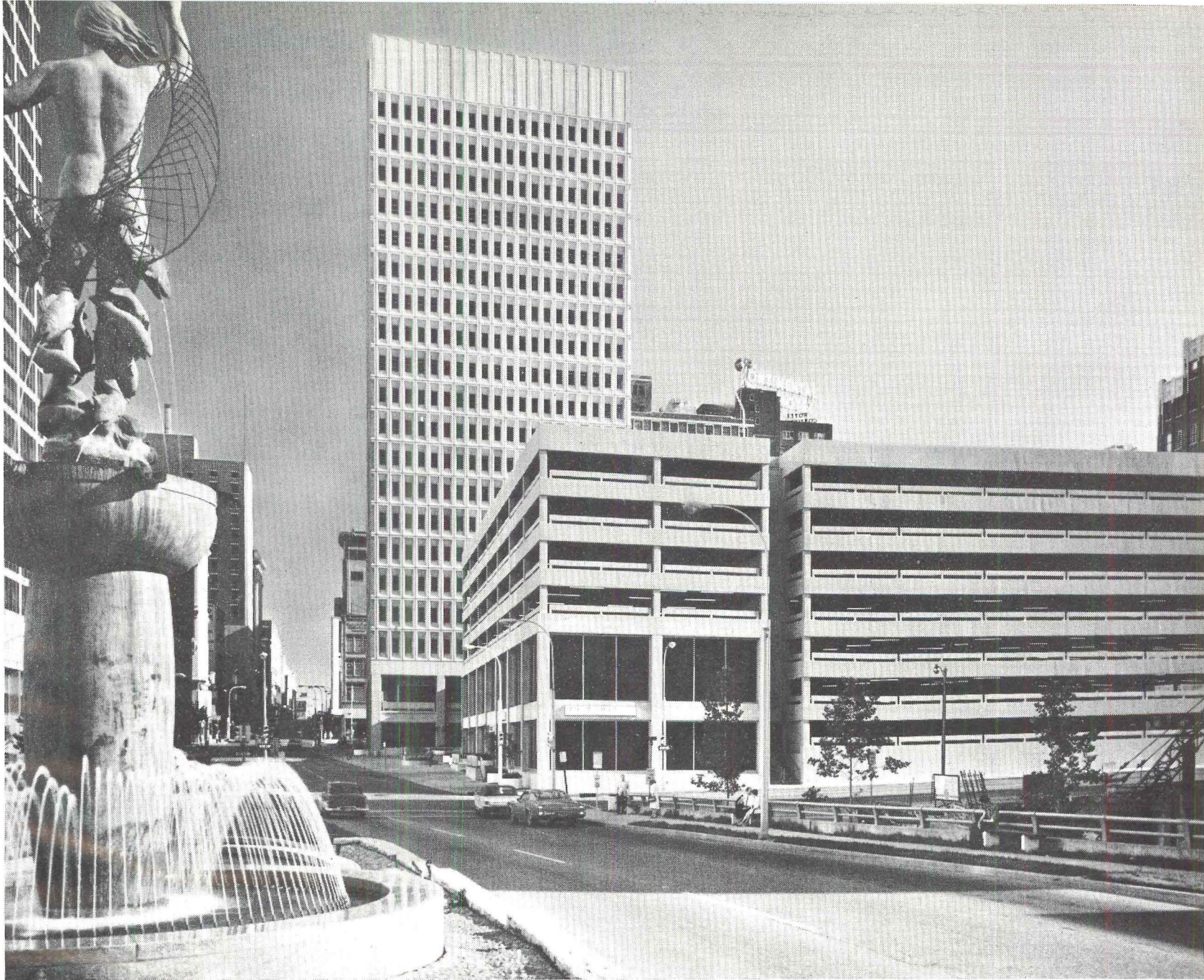
TenMain Center Office Building and Parking Facility, Kansas City, Mo. Monolithic reinforced concrete design/Robert P. Ingram, developer/ Charles Luckman Associates, architects/Marshall & Brown, associate architects/Howard, Needles, Tammen & Bergendoff, engineers/Winn-Senter Construction Company, general contractor/506,354 sq ft of standard Ceco steelform services/ 2,900 tons of fabricated reinforcing bars by Ceco.
