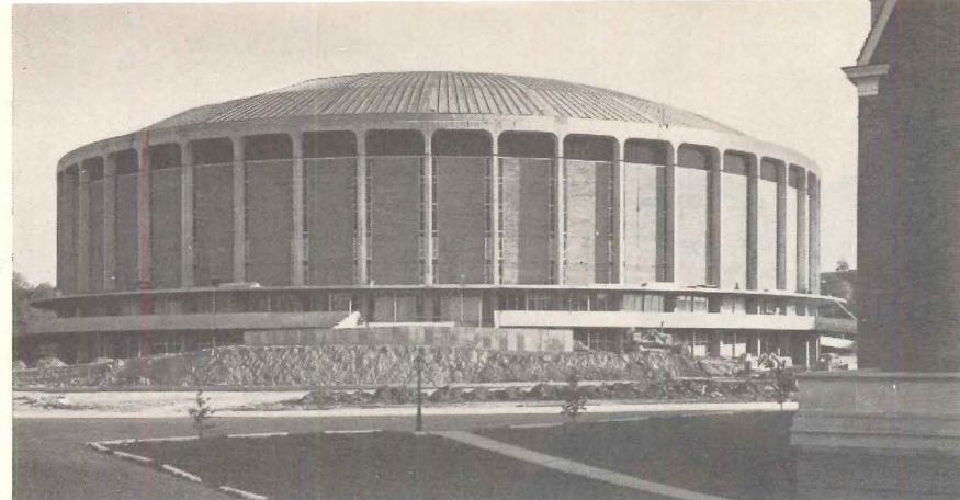
Ohio University Convocation Center, Athens, Ohio Architect: Brubaker & Brandt, Engineer: Fling & Eeman, Inc. Steelwork: Bristol Steel & Iron Works, Inc. General Contractor: Knowlton Construction Co.
