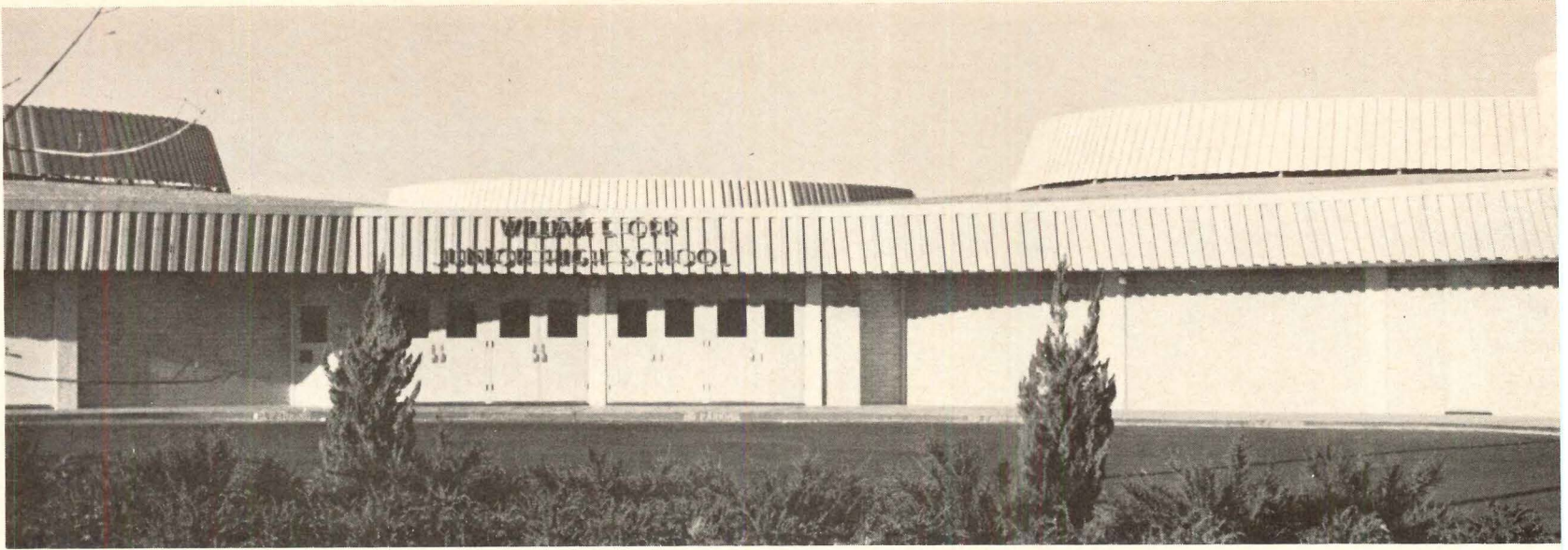
The low-profile Lennox DMS poses only a minimal screening problem. Example: The "pods" atop the William E. Orr Junior High School, Las Vegas, Nevada. Each conceals up to three DMS units. Architect: Zick and Sharp, in association with Shaver & Co. Engineer: Marvin Shafer.
