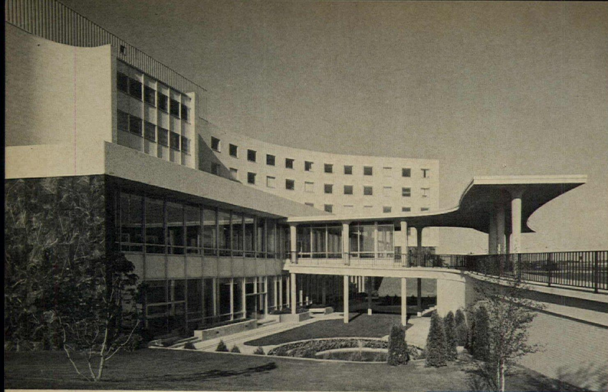
In the two-level base of Fairview Hospital, site conditions permit a glass-enclosed dining area overlooking a landscaped court at the lower level. A bridge from street level above the court gives access to the main lobby at the second level. An entrance for staff is on grade at the opposite side of the second level, where diagnostic and surgical services are located.
