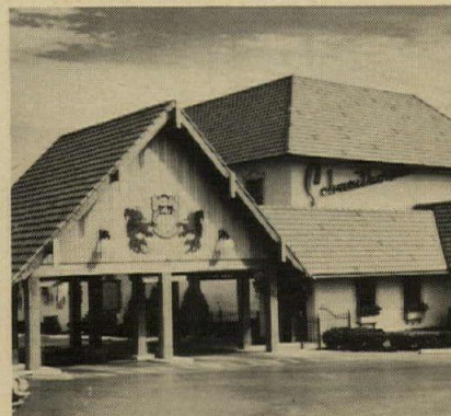
Schneithorst's Bavarian Inn. Gang-Nail flat roof trusses for mansard span 47 ft. and are 13½ ft. high. Trusses fabricated by Wood Tech Corp., Kirkwood, Mo.—Robert Elkington, AIA.
