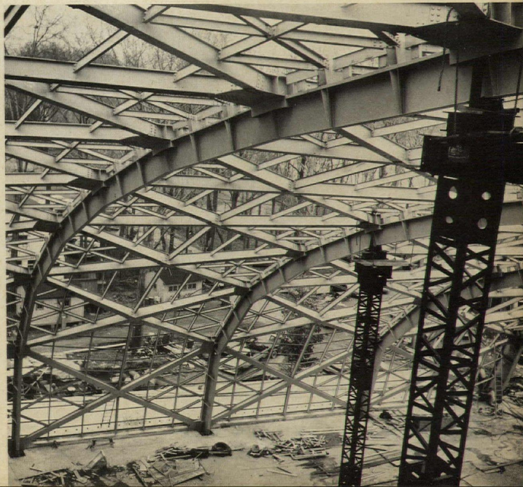
The unusual form of Princeton's new gym is shaped by a mammoth steel ribcage that spans 390 ft to house specialized functions and provide space for crowds of up to 10,000.
