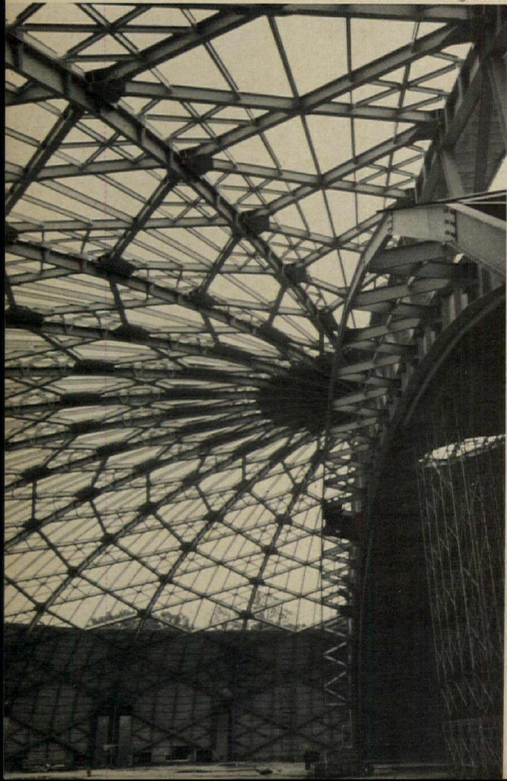
Intersection of the dome with an edge truss
