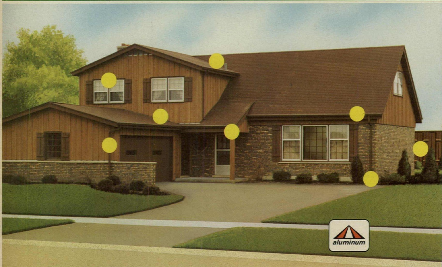
The "Concord": Pembroke Greens, Naperville, Ill.; as built by Harris Home Builders (land developers and home builders in Chicago area); Mr. William F. Harris
