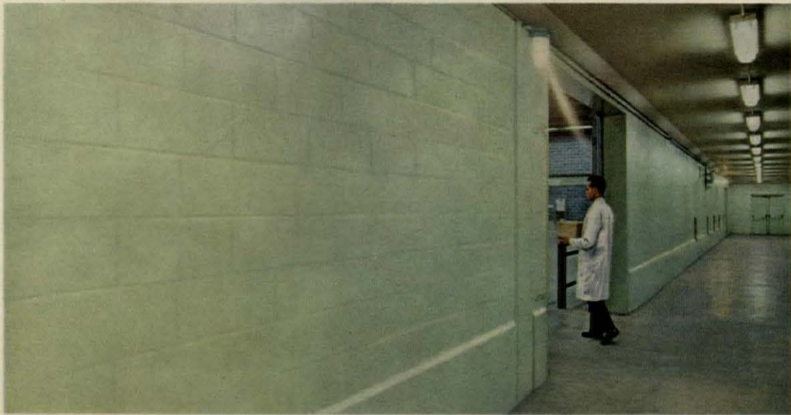
High-gloss, seamless Ply-Tile coating, based on Epon resin, prevents penetration of contaminants, cleans easily and quickly. A&P chose these coatings in yellow, blue, green and ivory for this food processing facility.
