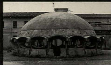
Balloon-formed concrete dome was erected at Columbia University last month by first laying reinforcement (spring-like coils plus bars) over an inflatable membrane which was tied to a perimeter ring. After concrete was placed, a different membrane was laid on top to help maintain evenness of the concrete as the balloon form was inflated. Photos left and right are of structure in Italy, illustrating openings cut out of the dome after construction.
