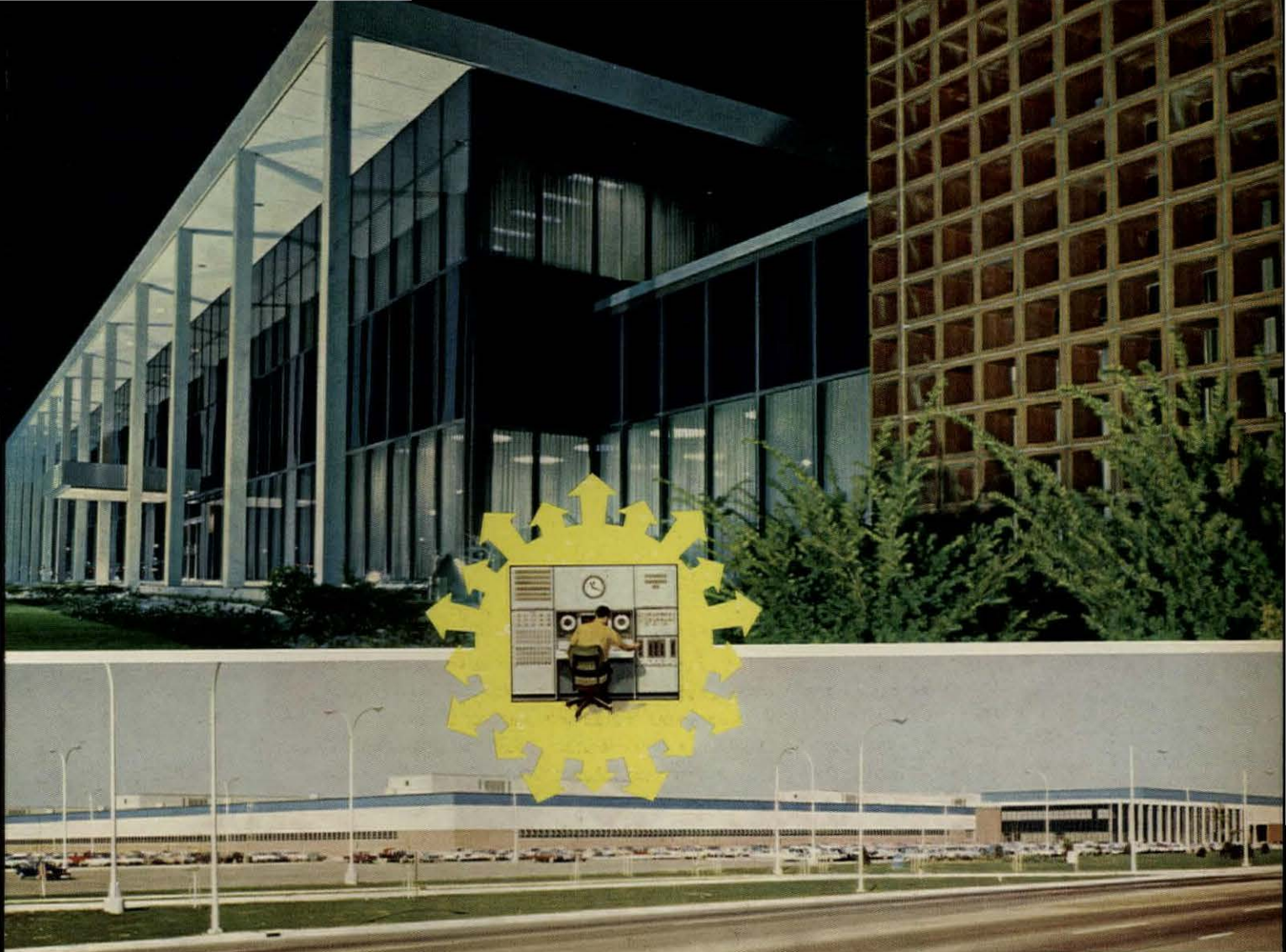
One man operates the Honeywell Control Center that starts, stops, adjusts, reveals, alarms, monitors, analyzes, and checks almost everything in an industrial plant. Shown here: Two views of 57-acre Chrysler Corporation Sterling Stamping Plant, Detroit, Michigan. Architects and Engineers: Giffels and Rossetti, Inc., Detroit.
