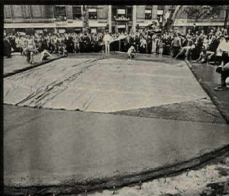
Balloon-formed concrete dome was erected at Columbia University last month by first laying reinforcement (spring-like coils plus bars) over an inflatable membrane which was tied to a perimeter ring. After concrete was placed, a different membrane was laid on top to help maintain evenness of the concrete as the balloon form was inflated. Photos left and right are of structure in Italy, illustrating openings cut out of the dome after construction.
