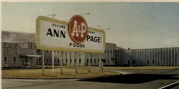
A&P food processing plant at Horseheads, N. Y., is the world's largest prestressed concrete building. Building perimeter is 1½ miles, and area under roof exceeds 1,500,000 square feet.
