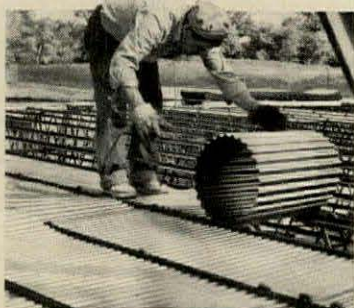
Deck can be easily placed by one man.
