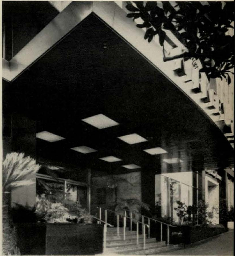
STAINLESS STEEL FASCIA brightens marquee, with stainless soffit. Kirkeby Center, Los Angeles, Calif. Architects: Claud Beelman and Associates, L. A. Fabricator: Construction Metal Work Co., L. A.
