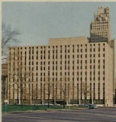
Southwestern Bell Telephone Office Building
