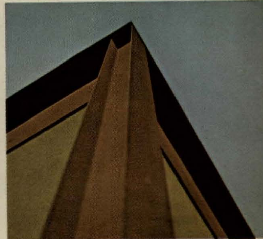
Photographs above taken after 12 months of weathering.
