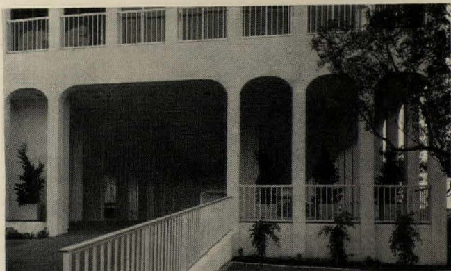
Seville Apartments, La Jolla, Calif. Architects: Neuhaus and Tayler, Austin, Texas; Assoc. Architects: Livingstone & Brown, AIA.
