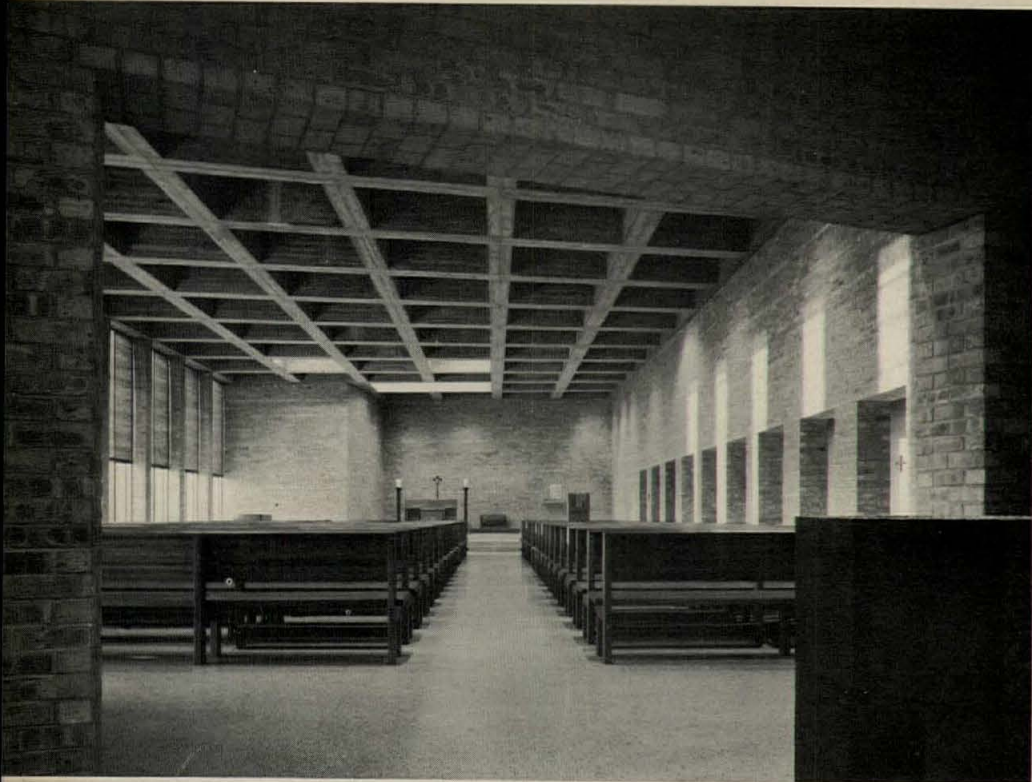
The chapel, above, and right in photo below, is a temporary one, which will be converted into a main dining hall when the academy is expanded in the future. (The bell tower shown in the rendering on the preceding page has not yet been constructed.) Exposed-brick walls and the unpainted-concrete ceiling give a considerable strength to the completely simple interior. Floors are terrazzo made with the same aggregate as the exterior walks.
