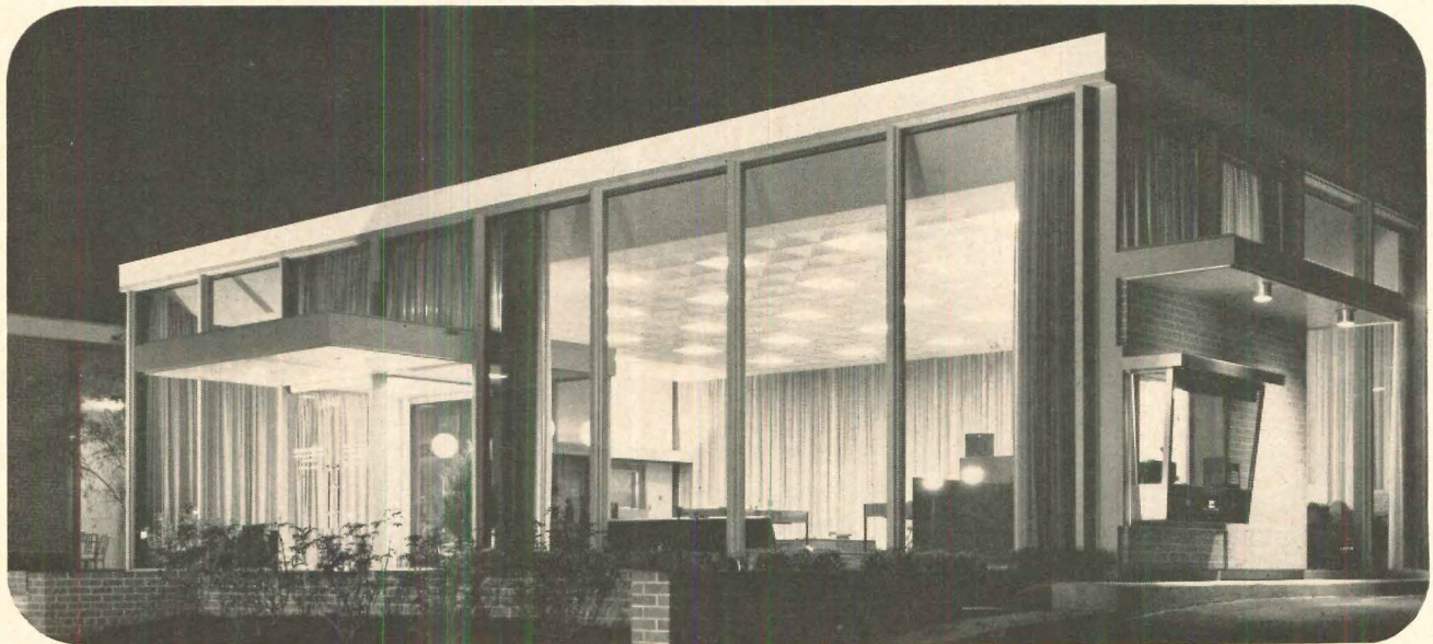
PARALLEL-O-GREY — Decatur Federal Savings & Loan, Decatur, Ga. Architect: Pope H. Fuller, Decatur. Glazing by Binswanger Glass Co., Atlanta.
