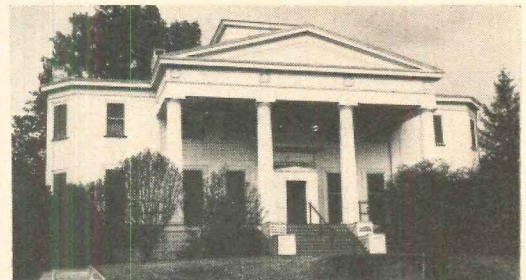
New York State Rehabilitation Hospital West Haverstraw, New York
