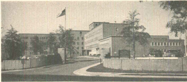
Maryland Veterans Administration Hospital
