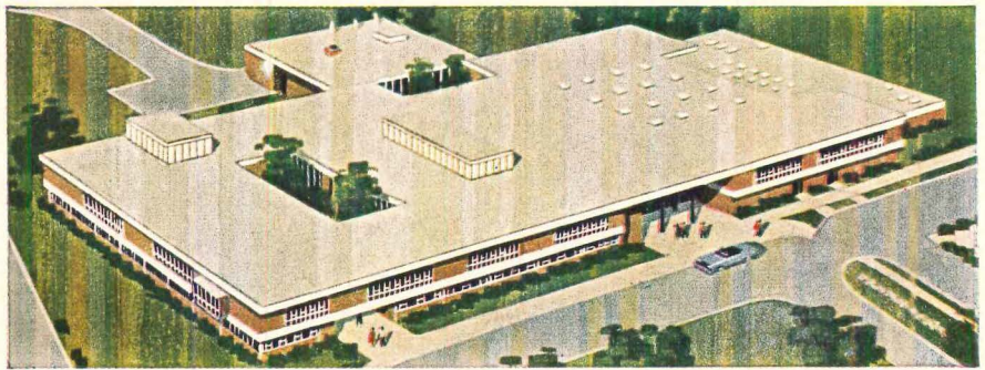
Another Barrett Bond Ply built-up roof. It's on this big Northern Highlands Regional High School, Allendale, N. J. Architects—The Perkins and Will Partnership. Builder—A. A. La Fountain, Inc.
