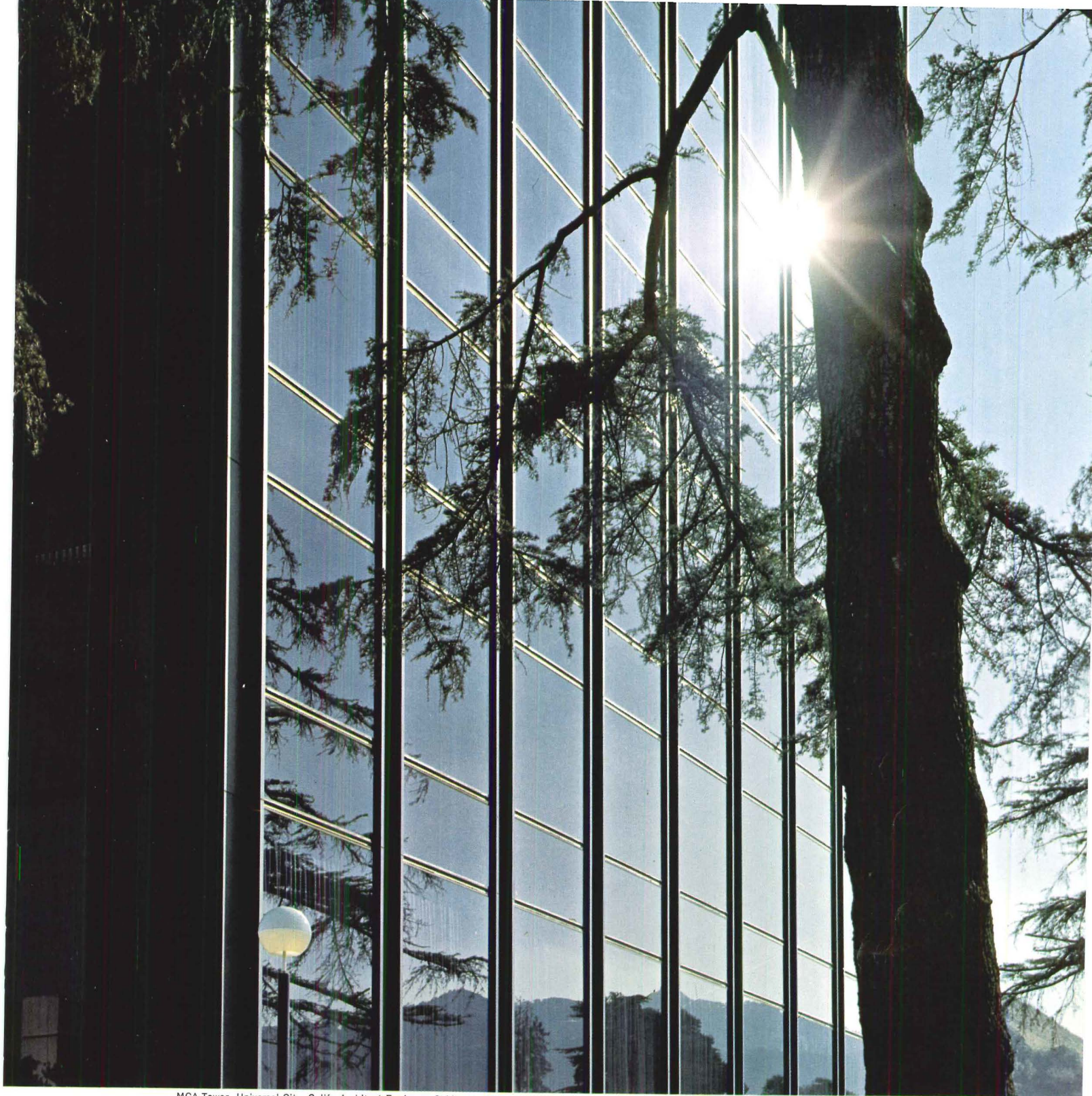
MCA Tower, Universal City, Calif.; Architect-Engineer: Skidmore, Owings & Merrill, San Francisco; KALCOLOR® aluminum fabricator: Fentron Industries, Inc.
