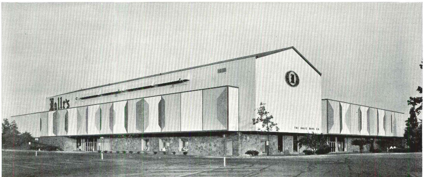
The Halle Bros. Co. Westgate Suburban Store, Greater Cleveland. One of eight department stores. Design Coordinator: Pierre Lalire. Planners and Designers: Raymond Loewy/William Snaith, Inc.; Architects: Fordyce & Hamby.
