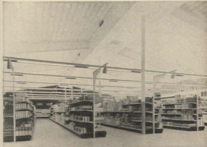
Tops Save-Cash Supermarket—Buffalo, New York Natural aluminum, two-lamp units in high ceiling supermarket.
