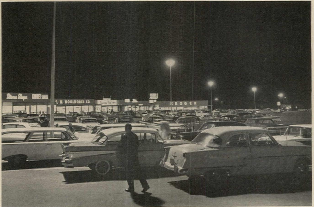
Relighting with eight 4000-watt Powerglow luminaires, mounted 35 feet high at 200-foot spacings, raised light level to an average of over two footcandles.
