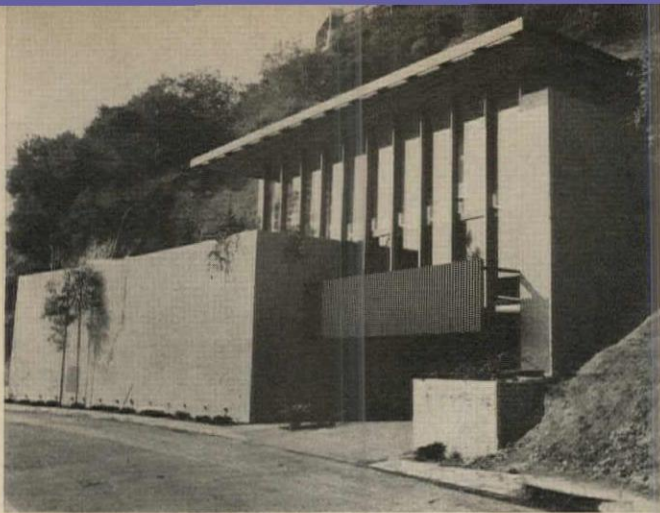
Residence of Mr. and Mrs. Carl Maston. Architect: Carl Maston; contractor: E. W. Hahn, Inc.; owner: Mr. and Mrs. Carl Maston
