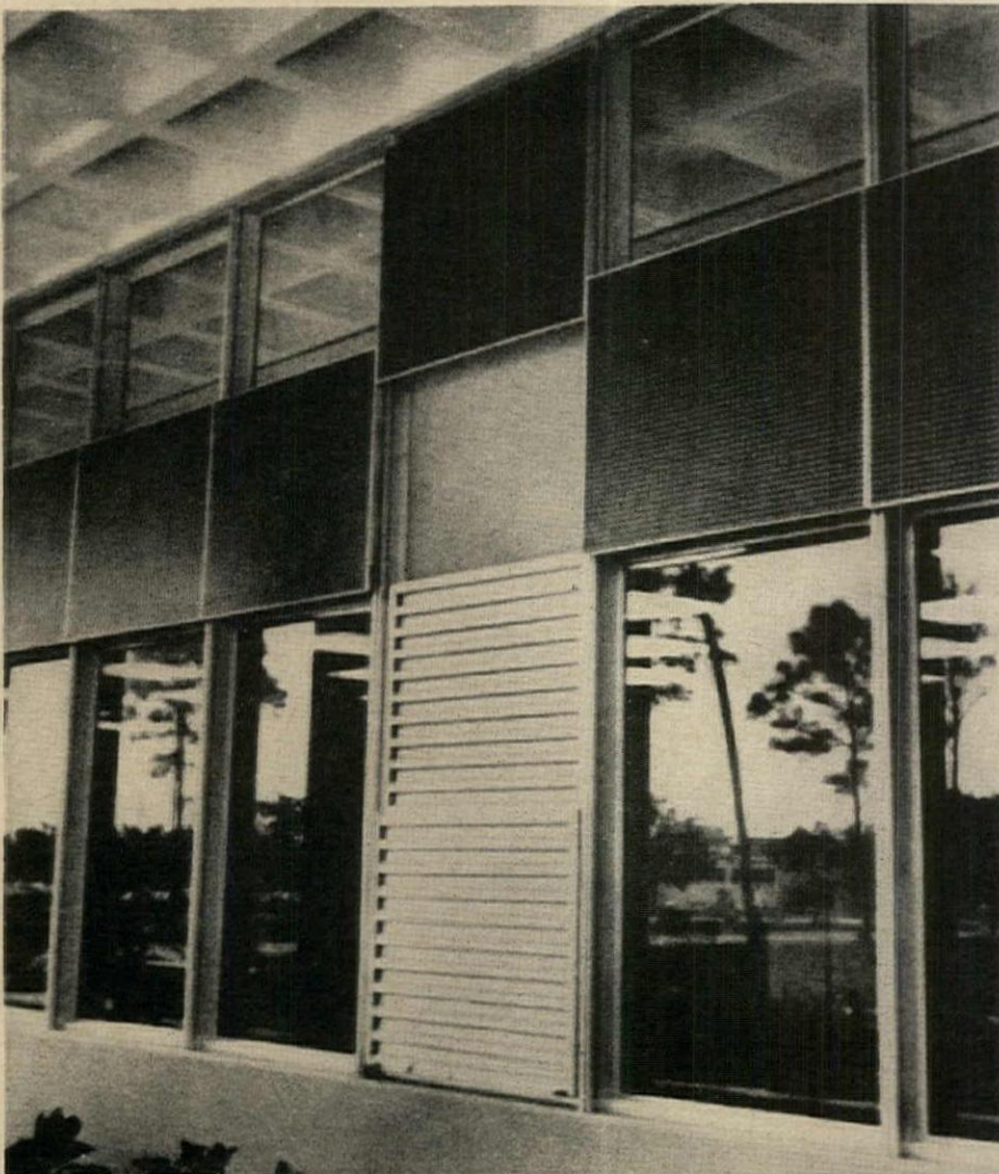
When a storm threatens, outer screen is pushed upward over clerestory window. Two inner screens of corrugated aluminum are then lowered in front of lower light
