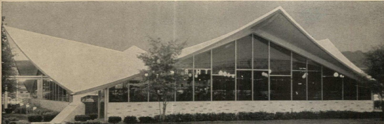
STEEL ROOF DECK FORMS HYPERBOLIC PARABOLOID
