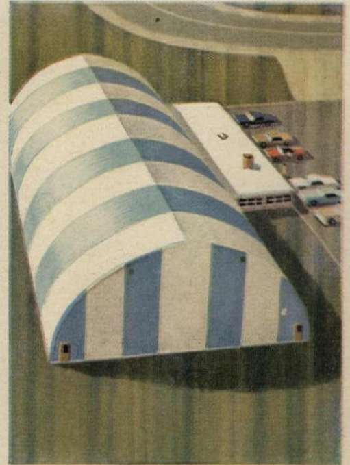
Three 48' sections of flexible 8 oz. Barrett Vinyl Panels were used to make each complete arch over the Philadelphia Aquatic School. This structure is 90' x 197' x 46' 6" high. Exterior steel cables anchor vinyl panels to building's frame.
