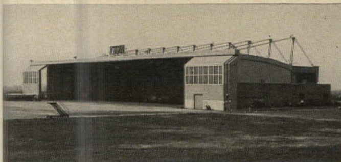
TWA Hangar, Philadelphia, Pa.
