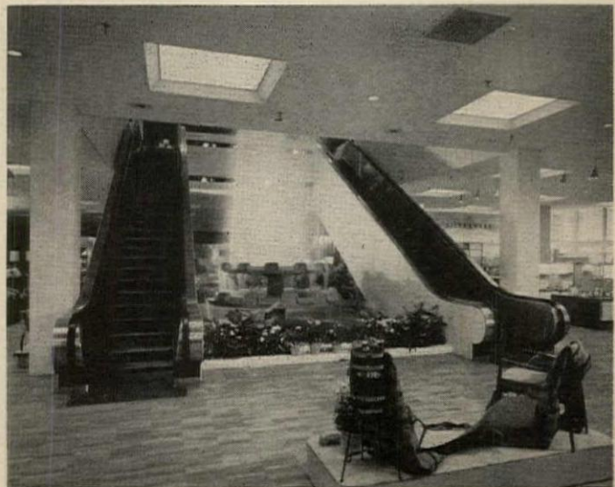
Figure 10. Parallel moving stairways in white marble are separated by a two-story fountain at Davison-Paxon, Lenox Square, Atlanta, providing an effective interior focal point, but at some sacrifice of merchandising space
