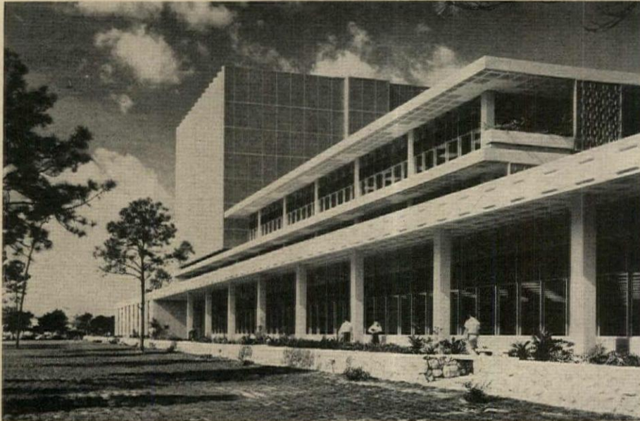
Each window has a nest of three hurricane screens installed between the main and clerestory lights. In closed position, only outer, stainless steel screen is seen
