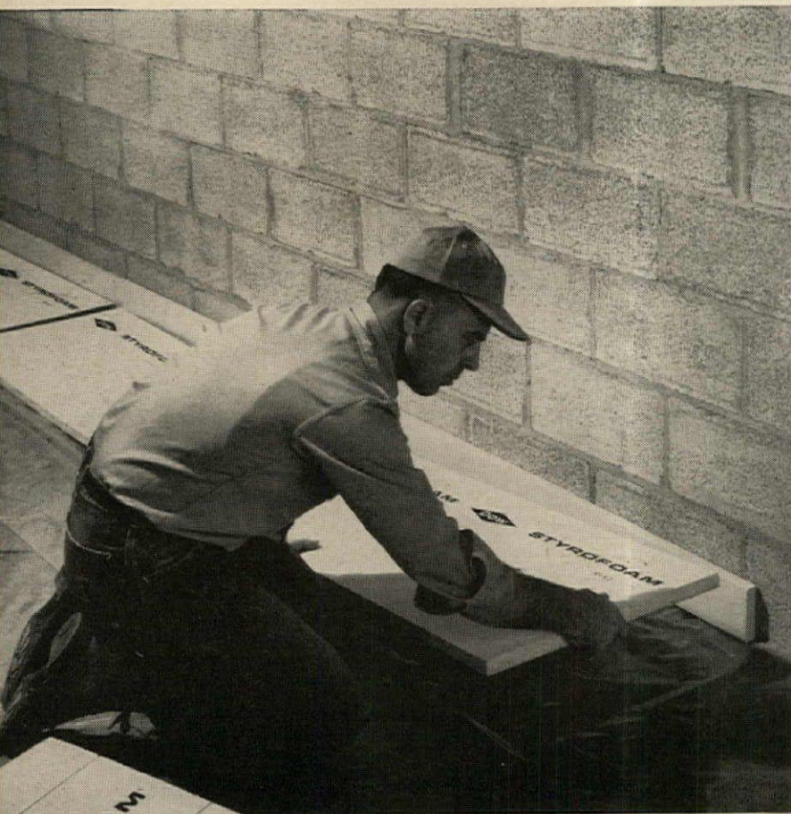
Remember Styrofoam for slabs and foundations.
