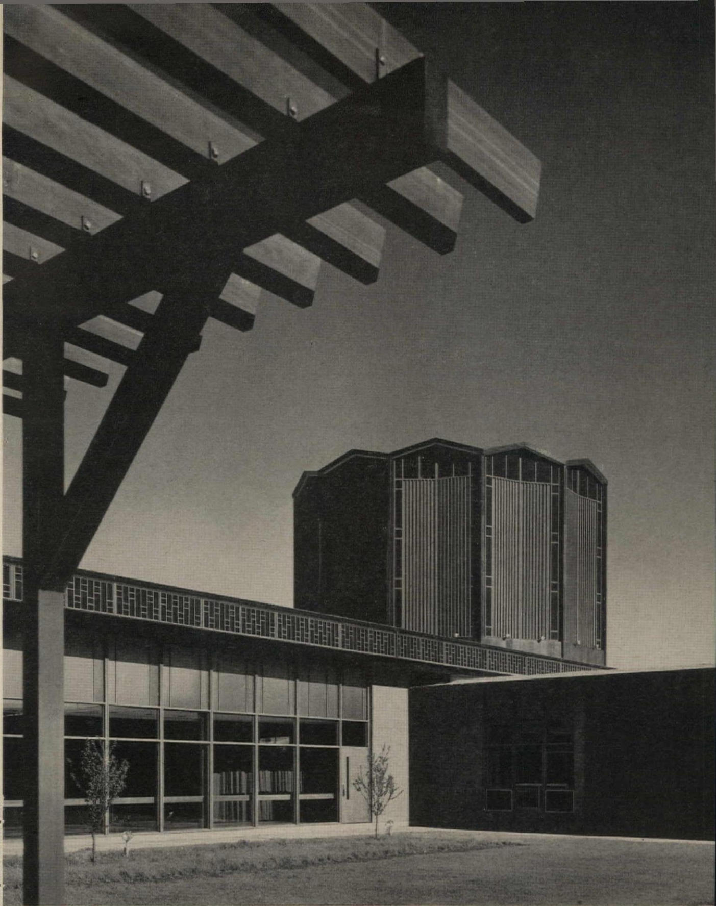
Dome and auditorium as seen from court
