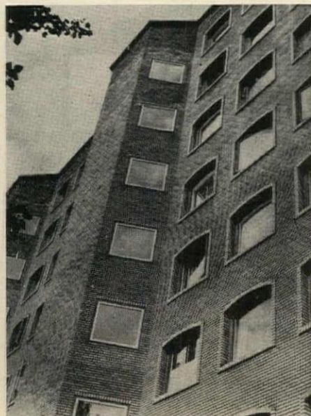
Built in 1943, this nine-story apartment building in Copenhagen is one of the earliest examples of multistory construction utilizing load bearing brick masonry. Regularly spaced cross walls are only 9 in. thick, stiffened by a central spine. Designed by Kay Fisker, C. F. Moller and Eske Kristensen
