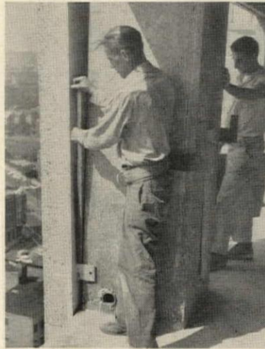
2 Mo-Sai panel is quickly and accurately bolted into position on the poured concrete supporting structure.
