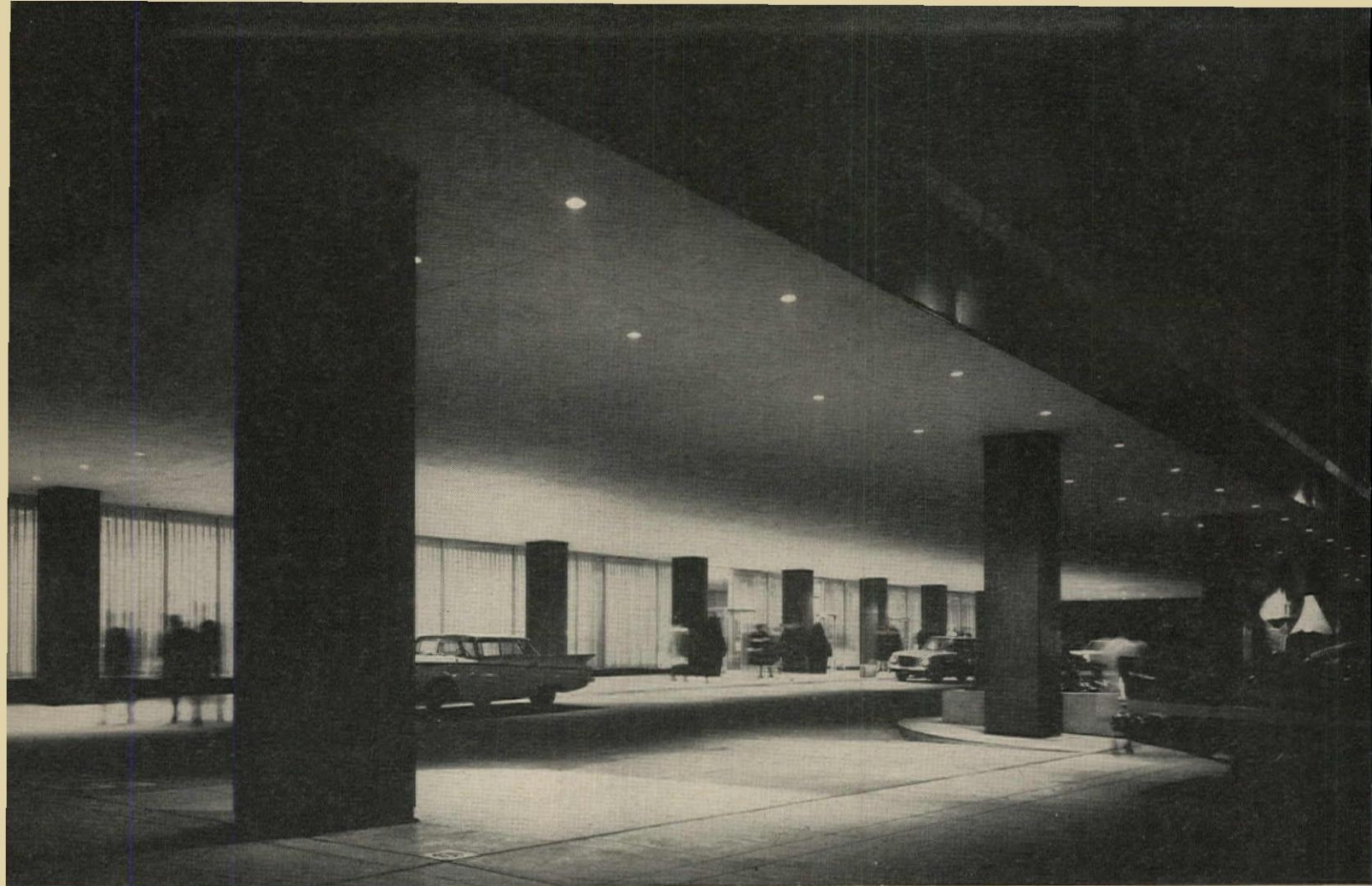
Drive-in entrance facilitates traffic flow, shelters patrons
