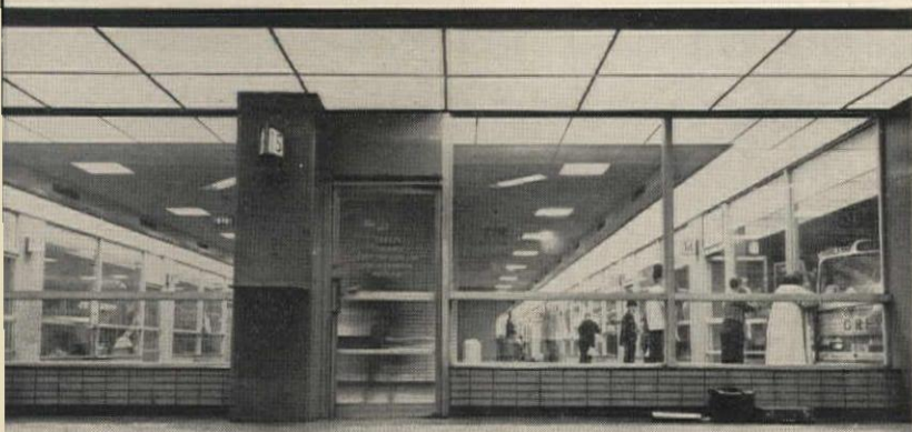
VIEW SHOWING BLOCK LONG ROWS OF LIGHTING LOUVERS
