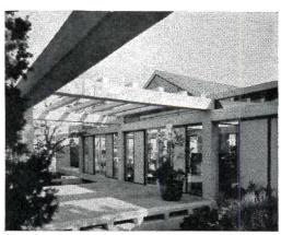
Broad entrance terrace, formed by one of the basic "Space Frame" units. Floor is of 2' x 16' precast concrete panels.
