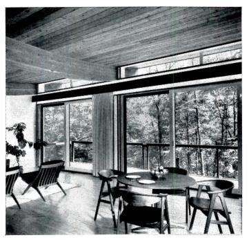
A room of fine wood furniture finds the narrow-planked flooring, tongue-and-groove ceiling, and laminated beams all in excellent taste. Floor-to-ceiling glass welcomes daylight as well as wood's variety of tones.
