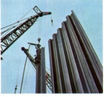
Just a stone's throw from Constitution Plaza, contractors pound home Bethlehem Steel sheet piling for substructures along I-84. Also on the job: Bethlehem H-piling, bracing, concrete reinforcing bars, and paving steels.
