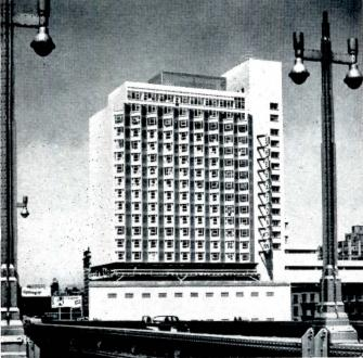
Sheraton Motor Inn, New York City, a 20-story reinforced concrete structure, is built in an L-shape, the façades angled so that each guest room has views. Containing 450 rooms, the new motor inn has a swimming pool on the twentieth floor and a four-level ramp garage for 300 cars. Architects were Morris Lapidus, Harle and Liebman. Builder was Louis J. Glickman
