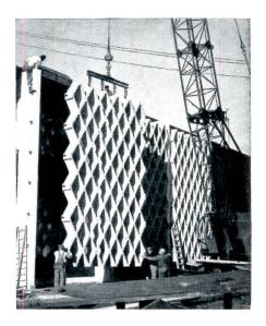
On the exterior, the lab building has a large precast sun screen on the east and west; fin-like baffles protect the other two sides. All are white to contrast with the brown brick walls. The screen is made up of 46 panels, each weighing 5½ tons and measuring 22 ft high, 14½ ft wide and 16 in. deep.
