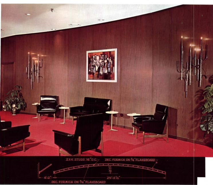
A decorative non-loadbearing wall can be erected quickly and inexpensively to any shape with Formica laminated plastic.
