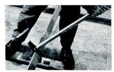
Switches and outlets can be located wherever needed, in General Electric Flexway Wiring. Devices fit onto a base channel, and the spaces between them are closed with raceway covers, easily cut to length with a special tool.
