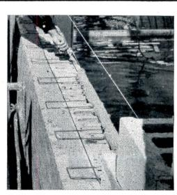
Made of all 3/16" wire or all #9 wire. Made in 12 foot lengths with 4" wide box ties 16" O.C. (9 ties per length). Available finish: Galvanized box ties with brite basic side rods; all mill galvanized wire; hot-dipped galvanized after fabrication.
