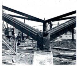
Half-round pipes on edge beams are used for welding attachment of roof
