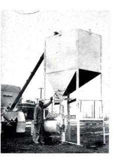
hand shoveling, separate deliveries of materials, time lost in thawing sand piles, and the need to protect materials from the elements. *Instant Crete Corp.*, *Linden*, *N.J.*
