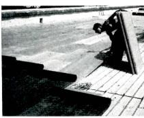
covered with a coated base sheet. The roof is completed by mopping top of coated base sheet with asphalt and placing standard roofing felt in conventional manner. The insulating foam is light weight and is manufactured in two by four ft lengths in five thicknesses. Dow Chemica Co., Midland, Mich.
