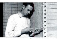
Keywall "tails" to be tiedin later. You can appreciate this advantage when continuous reinforcement is needed, even though some wall sections must be left unfinished for other work. Only Keywall is flexible enough to accommodate variations in mortar joint levels,
