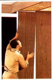
For fast installation, Marlite Random Planks ( $^{1}/_{4}''$  x 16" x 8') are tongued and grooved—assure a better finished job.
