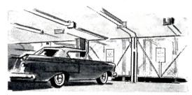
Automatically-operated, upward-acting, expandedmetal gates by "OVERHEAD DOOR" are used in this pigeon-hole parking structure at Columbus, Ohio. Representing the newest in car-park automation, this driverless "file system" depends on The "OVERHEAD DOOR" for swift, automatic handling.
