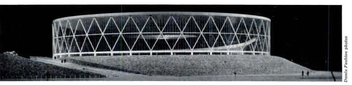
Arena roof, 420 ft in diameter, is of precast concrete T's placed in three rings
