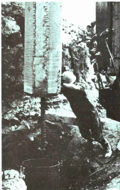
Splicing an 18-in. octagonal prestressed, precast concrete pile
