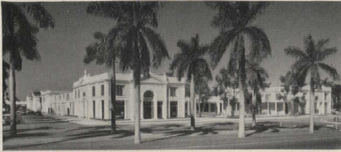
Approximately 40,000 square feet interior and 20,000 square feet exterior terrazzo made with Trinity White portland cement is in the Royal Poinciana Shopping Center, Palm Beach, Florida. John L. Wolk & Associates, Palm Beach, Architects; terrazzo by E. R. Anderson & Co., West Palm Beach.
