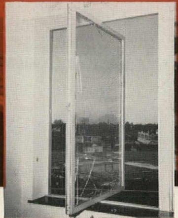
Weatherstrip still intact, this Baptist Memorial hospital window, typical of the Adlake reversibles exposed to flame, retained its glass in spite of temperatures which reached 1200° plus for more than thirty minutes. Unretouched photo reveals how glass cracked but did not shatter.
