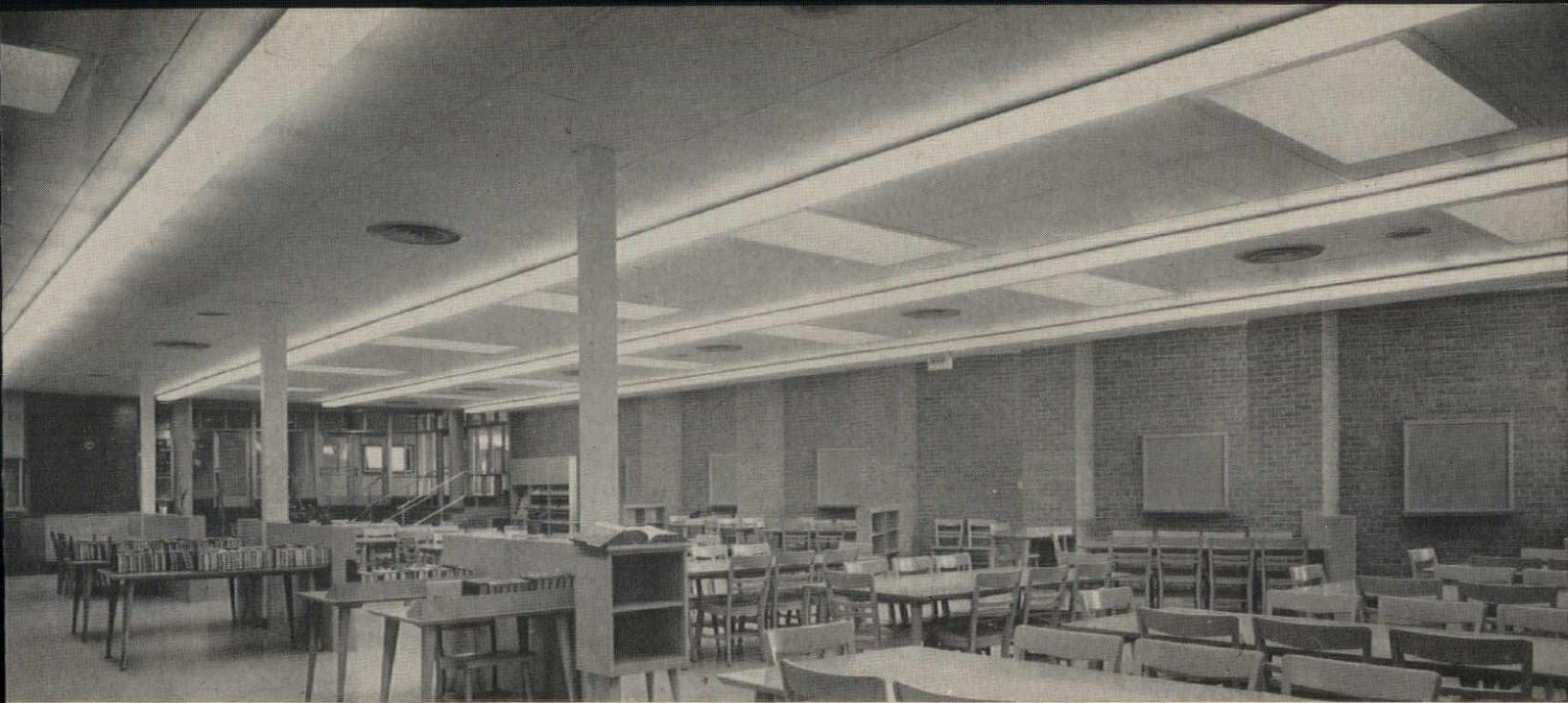
Superb Day-Brite Holiday fixtures maintain a minimum lighting level of 70 footcandles.
