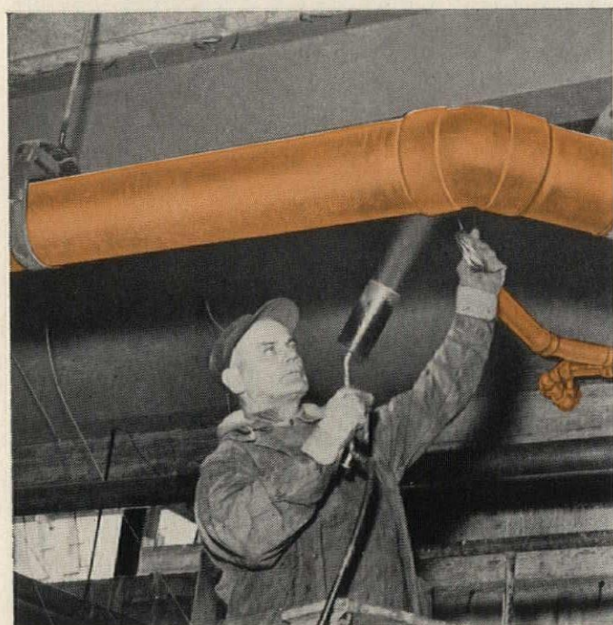
MAKING A SOLDER JOINT on an 8-inch copper soil and waste line — the largest size used in the drainage system. Solder-joint connections are one of the important reasons why copper tube systems are so much easier and faster to install.
