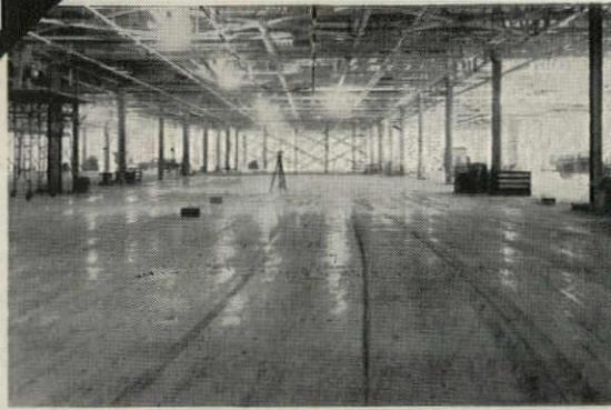
Western Electric Plant, Columbus, Ohio
