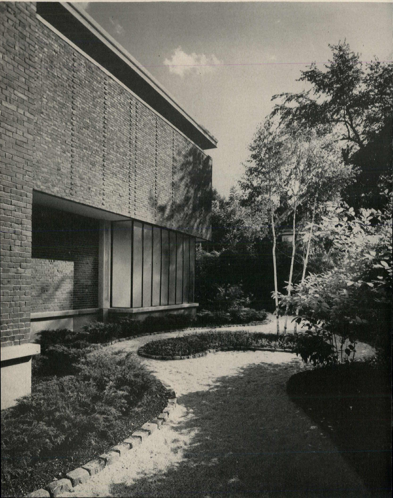
Two level tryout room exterior
