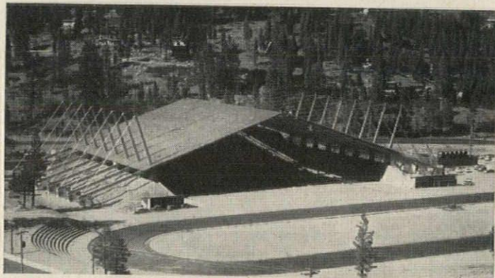
Looking like a giant wigwam, this unusual structure can shelter some 8,000 winter sports enthusiasts in relative warmth and comfort.
