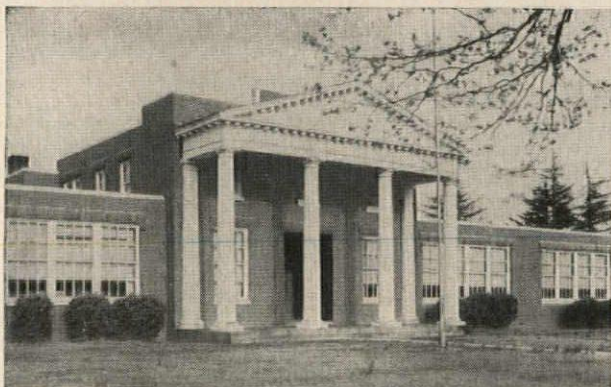
Applied 28 years ago—still in service. The Accomac Elementary School, Accomac, Virginia—a typical example of economy and durability with RUBEROID roofing. This Special Bitumen job, done in 1932, is a four ply 15# Asphalt Felt, Bitumen and gravel surface on one inch of insulation.
