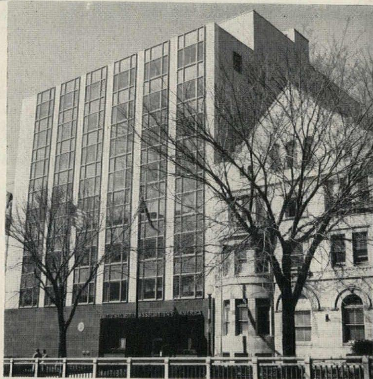
National Rifle Association of America. New building is heated throughout with Lo-Blast Gas Burners, installed on the roof to save valuable space.
