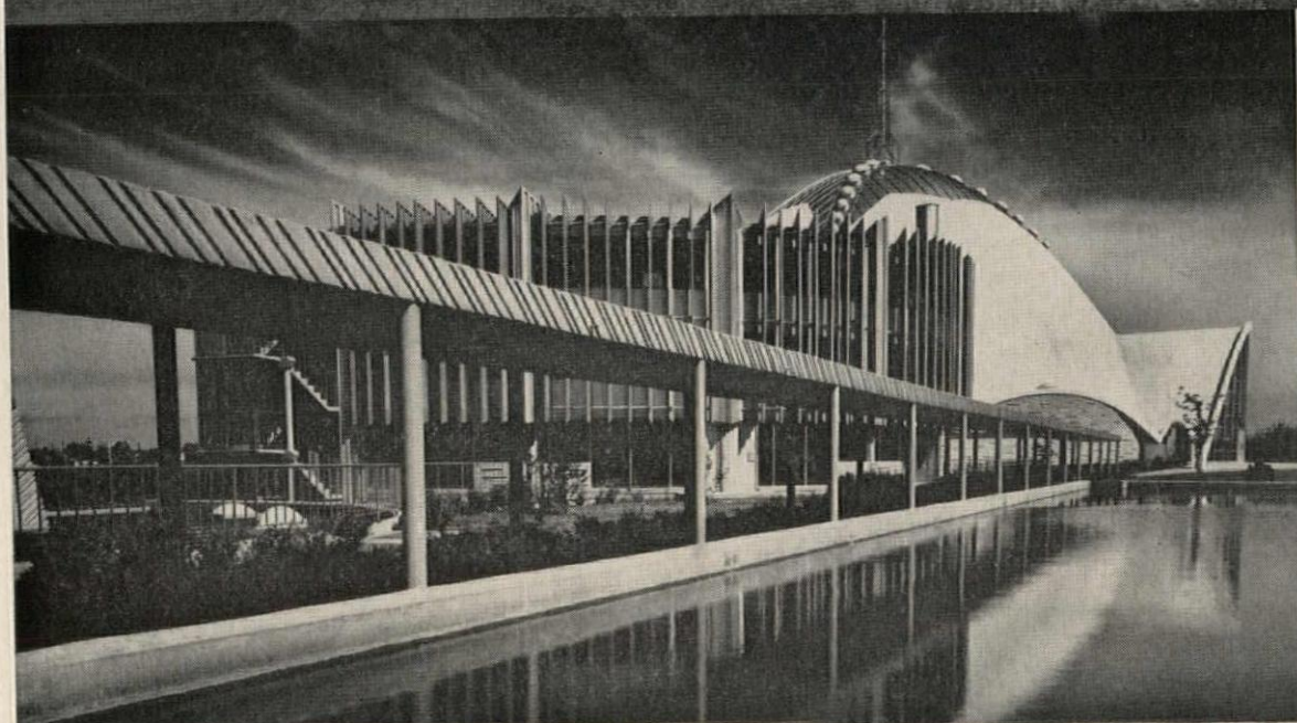
First Christian Church of Tomorrow, Oklahoma City, Oklahoma. Ceco Curtainwalls of 1½" intermediate projected steel windows with aluminum panels; Connor & Pojezny, architects; Frederickson & Parks, Inc., contractors.
