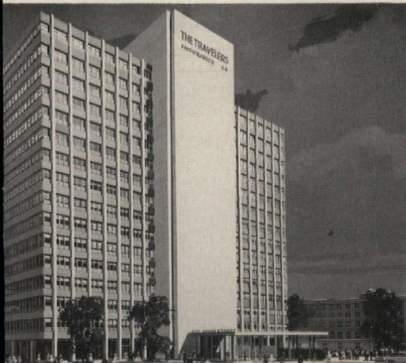
Sprinkler System and Stand-Pipe Fire Lines in Travelers Insurance Boston building are durable steel pipe. Savings in initial and installation costs were considerable; insurance premiums were less with steel pipe fire protection systems on guard throughout the structure.
