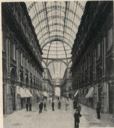
Galleria Vittorio Emanuele, Milan; Mengoni, architect
