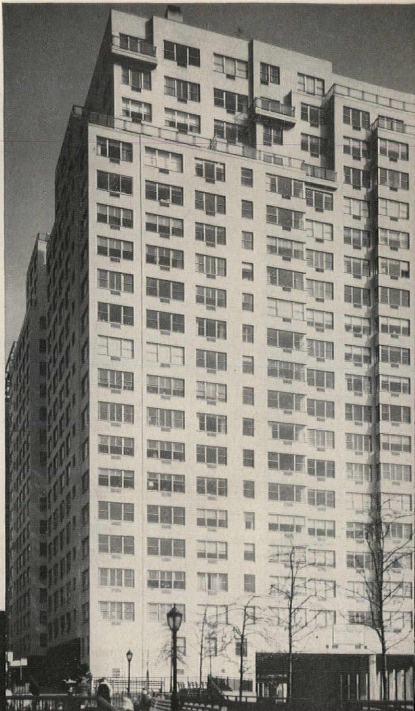
Apartment Building, Cannon Point South, New York, N.Y. Ceco series 60 aluminum double-hung windows: Paul Resnick, Harry F. Green, architects; Blitman & Tischler, supervising engineers.
