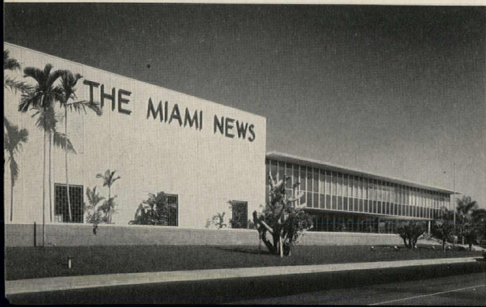
MIAMI DAILY NEWS, INC., Miami, Fla. Architects-Engineers —Weed Russell Johnson Associates. Contractors —C. F. Wheeler, Builder, Inc. Rotary Oildraulic Elevators sold and installed by Miami Elevator Co.
