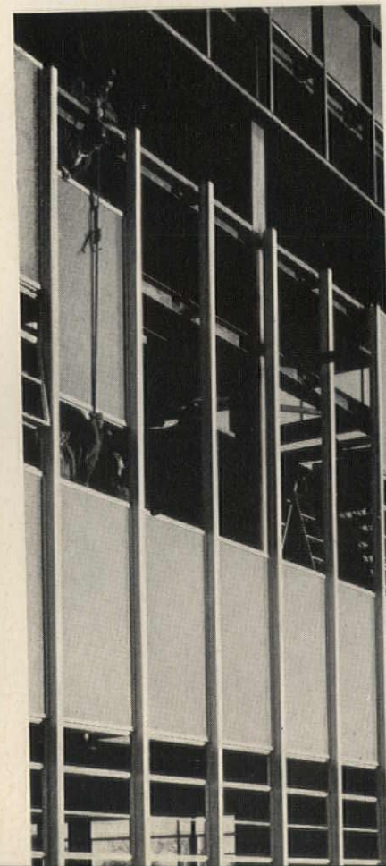
STURDY AND STREAMLINED. Laminated-polyester entrance-canopy support has done its job perfectly... with no observable distortion, deflection, or discoloration.
