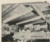
Holiday Inn Motel, Springfield, Illinois, constructed with Rilco laminated wood beams up to 31' 9" in length. Architect: G. Wayne Hopper. Contractor: General Contractor, Inc., Springfield.
