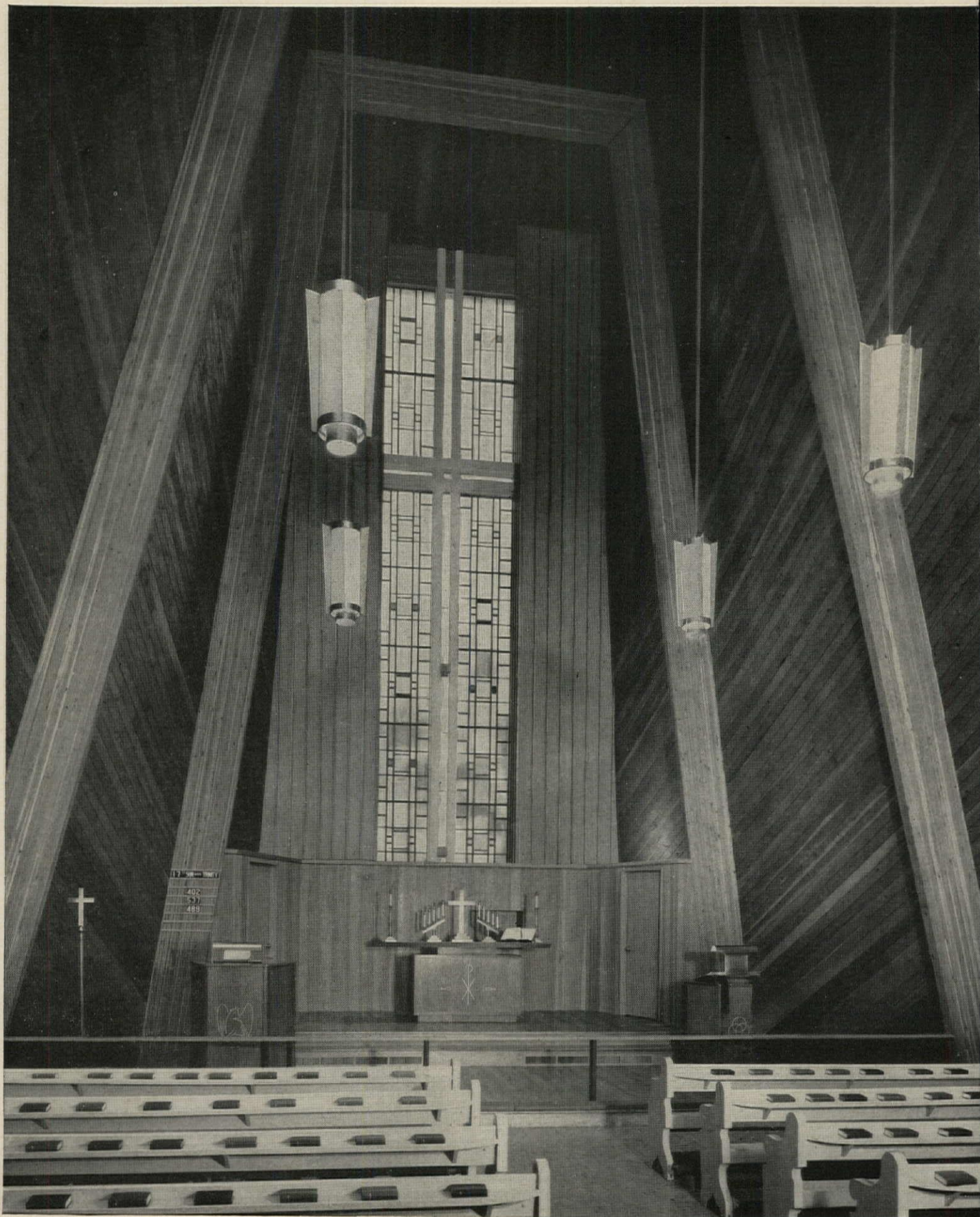
Allowing wood to function structurally and decoratively helped realize significant economies in the construction of this modern church. These dramatic supporting members are 2x6's over laminated arches. Sargent, Webster, Crenshaw and Folley, architects.
