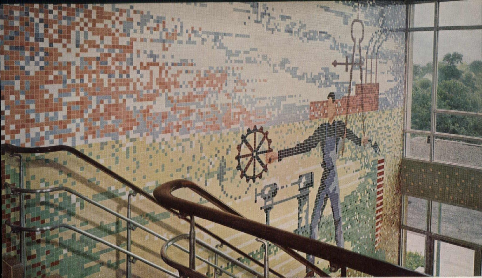
Williamson Free School of Mechanical Trades, Media, Pa. Wall Mural in 1½" Tile Gems® in 27 Bright, Matte, Crystalline, Decorator and Special Colors. Interior Spandrel: 1½" Tile Gems® in 76 Sage Gray, and 58 Vellum. Architect: Massena & duPont, Inc., Edward C. Cooper, Associate. Tile Contractor: United Marble Co., Inc. Color Plate 420.
