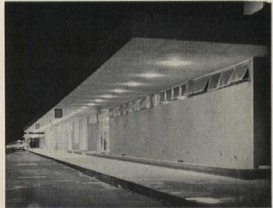
FORT LAUDERDALE AIRPORT Kirlin wide angle lenses light both vertical and horizontal surfaces. Note how car in background stands out
