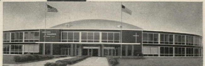
Beautiful and modern, the Church of Tomorrow near Akron, Ohio, features Haskelite panels with fiberglass reinforced polyester faces, cement asbestos interbands and foamed polystyrene core. Architect: A. L. Salzman, Chicago.
