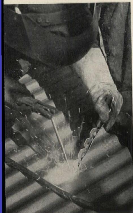
Exclusive Fab-Form Welding Washer Stick reduces installation time. After the end washer on the stick is bent up, the welder makes a plug weld and snaps off the washer. Then mesh is installed and slab is poured.
