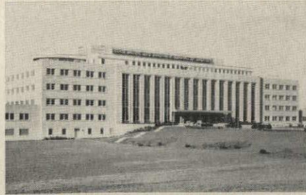
$9,000,000-plus home of State Mutual Life Assurance Company of America, Worcester, Mass. Arch: Hoyle, Doran & Berry. Elect. Eng: Thompson Engineering Co. Elect. Cont: Coghlin's, Inc.
