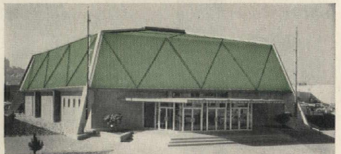
Memorial Building of the International Longshoremen's and Warehousemen's Union, San Francisco. ARCHITECT: Henry Hill, San Francisco. The dome is sheathed with about 18,000 sq. ft. of Economy Copper Roofing installed by Fire Protection Products Co., San Francisco.
