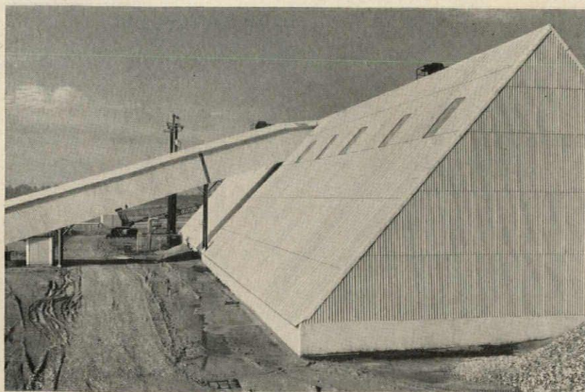
Roof windows of corrugated plastic fit neatly into Corrugated ASBESTONE "400".
