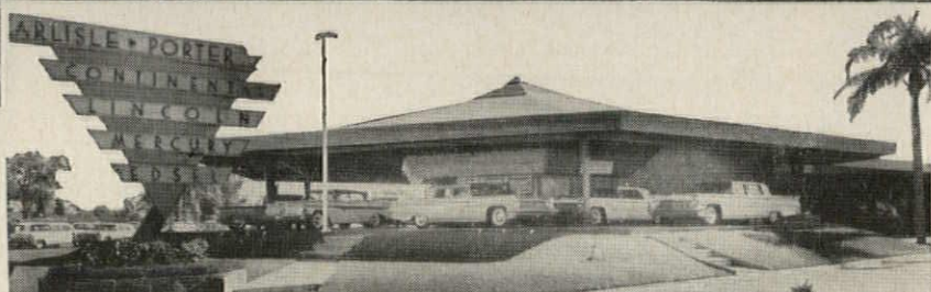
"A landmark in this area," says H. H. Carlisle of his firm's recently constructed Rilco building in Clearwater, Fla. Architect: John Randall McDonald, AIA, Indian Rocks Beach, Fla.
