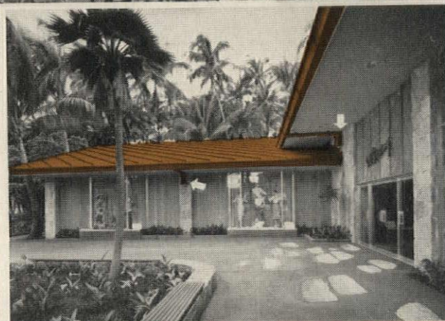
ENTRANCE TO THE fabulous McInerny Waikiki Store. Known as "The Jewel of the Pacific," it is one of the show places of the world, and is in Honolulu, Hawaii. Note how copper gutters blend into roof line; also unique treatment of down spouts (arrows).
