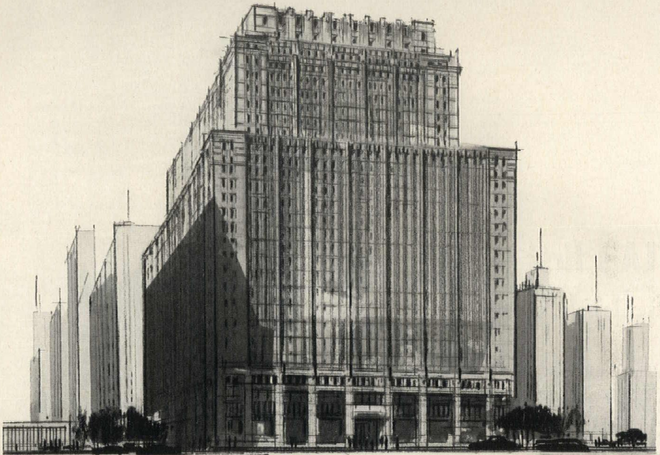
2 Park Avenue, New York City. Consulting Engineers: Sears and Kopf; Mechanical Contractor: Kennedy-Scheidel-Young, Inc.; Electrical Contractor: Theodore Kaish, Inc.
