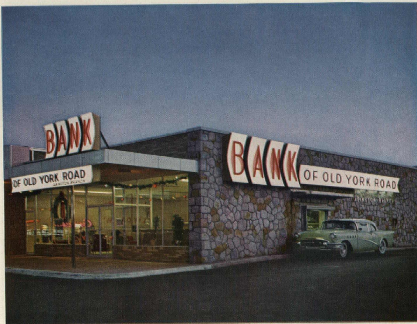
PLEXIGLAS letters and modular background panels at Bank of Old York Road, Abington, Pa. Architects: Haag & d'Entremont
