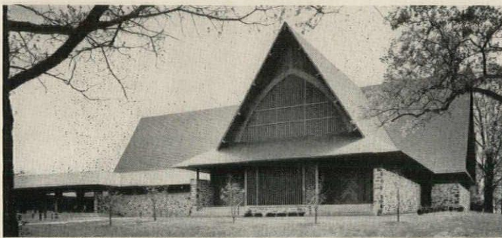
The Church of the Redeemer, Baltimore. Architect: Pietro Beluschi, F.A.I.A., and Associated architects: Rogers, Taliaferro & Lamb. Engineers: Henry Adams, Inc. Owner: The Church of the Redeemer. General contractor: Consolidated Engineering Company, Inc.
