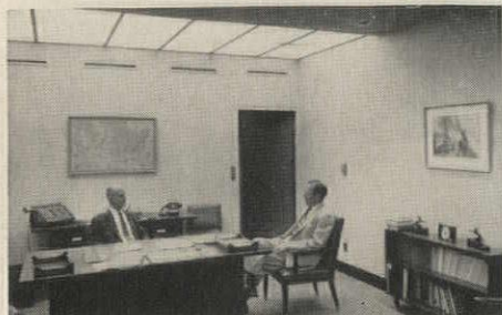
Solid section in illuminated office ceiling permits flexibility of lighting — 6 G-E switches control warm and cool fluorescent and downlight combinations to please any occupant.
