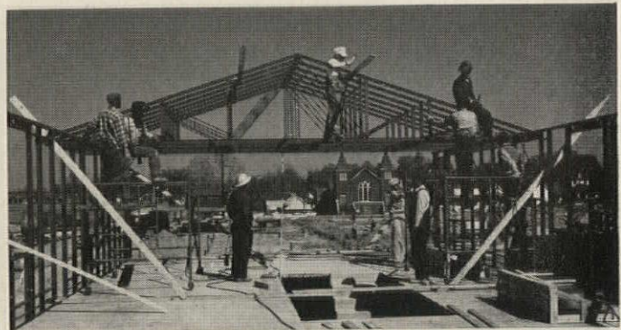
Every five minutes, workers lifted 31' trusses weighing only 140 pounds into place—including welding to the top channel of the load-bearing wall.
