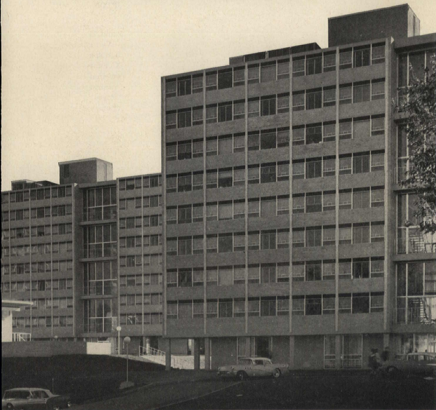
Architect: Hellmuth, Obata and Kassabaum, St. Louis, Mo. Contractor: D. C. Bass & Sons Construction Co., Bass Bldg., Enid, Okla.
