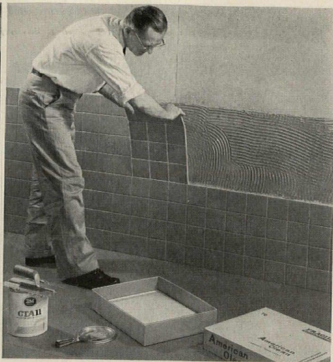
Master-Set sheets go from carton to wall in one motion with no soaking needed—can be installed with adhesives, thin-set mortar, or conventional cement mortar with self-curing bond coat.
