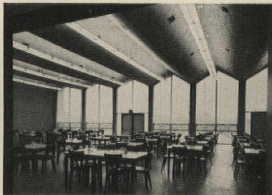
Main dining room, showing exposed concrete roof structure.
